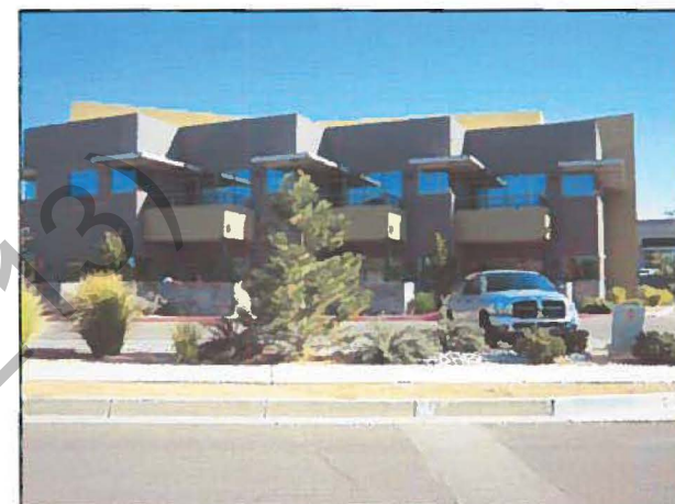
This building is divided into vertical segments, reducing the mass and providing interest from the street view.
