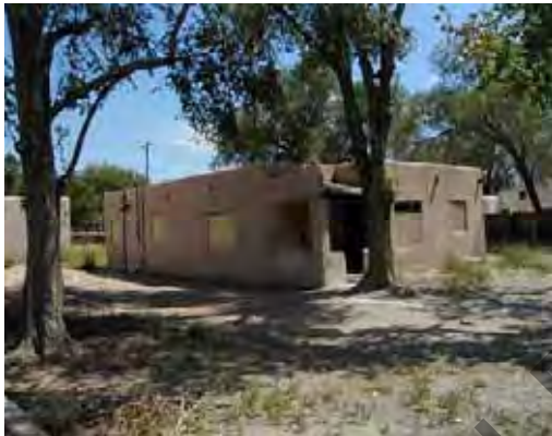
(12th and Major before demolition)
