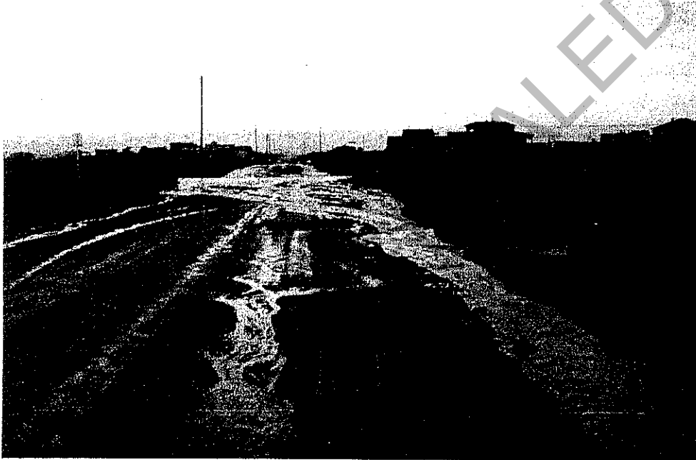
Figure 3 - Diversion caused by road crossing of arroyo
