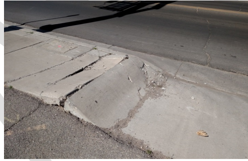
Buckling sidewalk and pavement
