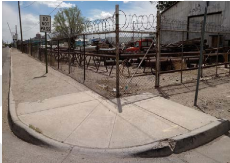
Accessible ramp with no connecting sidewalk
