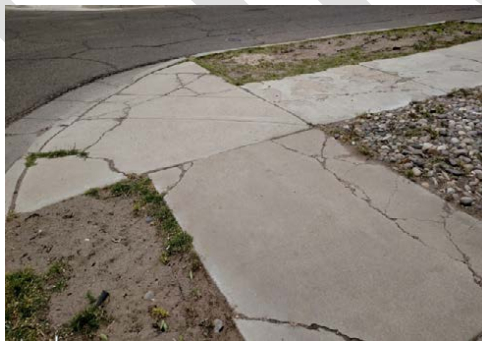
Crumbling sidewalk from shifting land underneath
