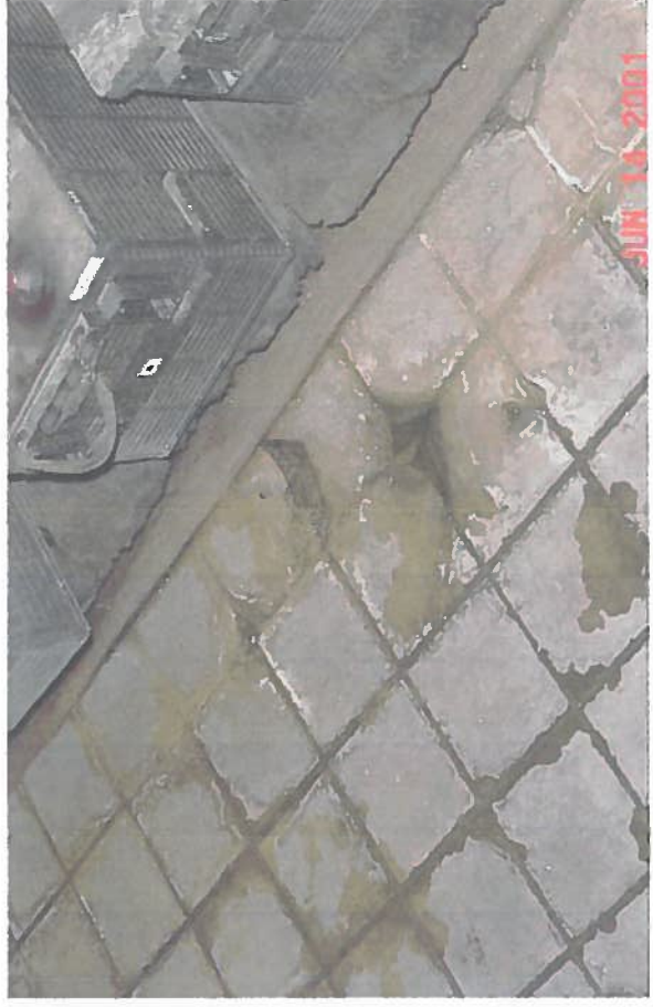
Photograph 12. Close up view of the acid corrosion on the floor in the battery storage room.
