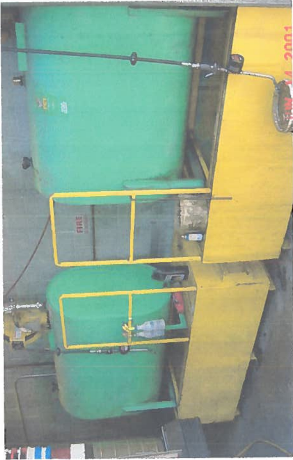
Photograph 13. View of the ASTs containing new oil in the shop.
