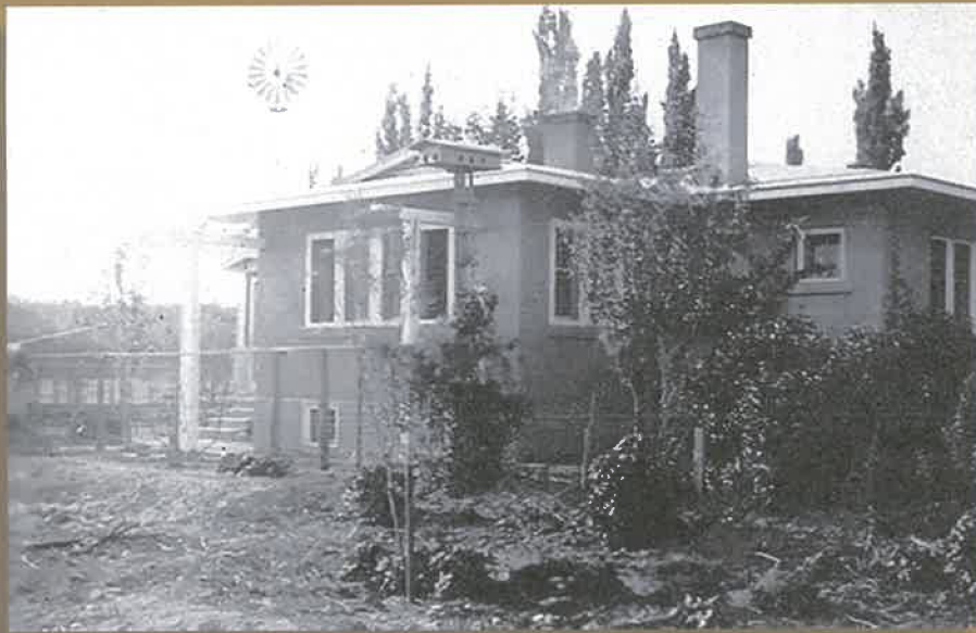
Leopold House looking northwest
