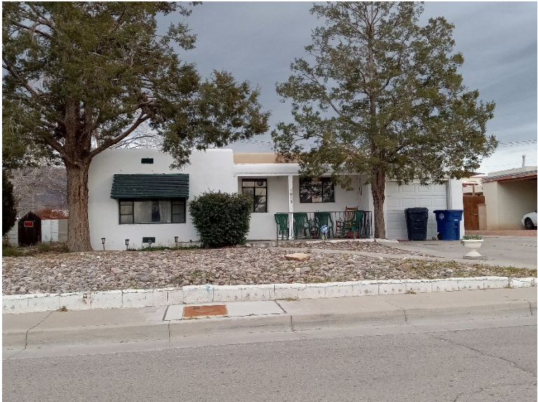
Figure 8: East End Addition Properties
