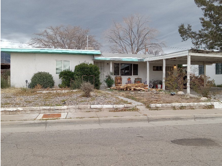
Figure 7: East End Addition Properties
