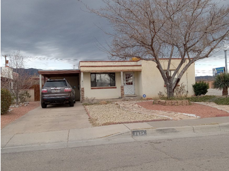
Figure 9: East End Addition Properties
