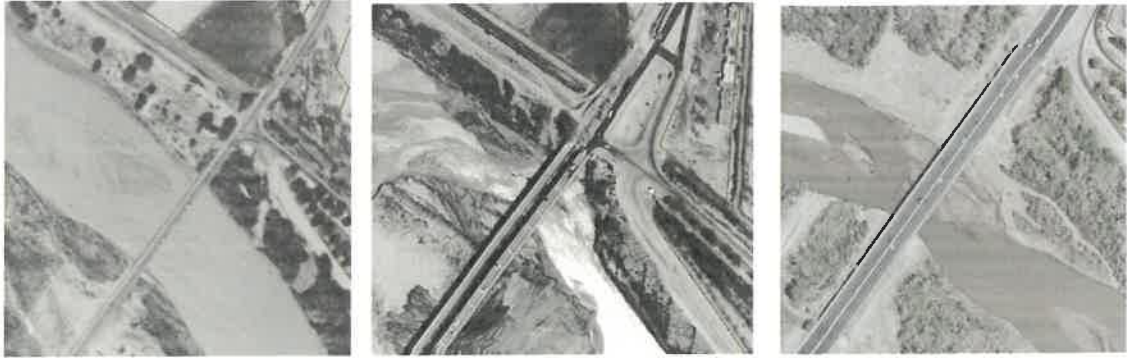
Figure 2:Central Ave Bridge crossing 1930, 1953, 1983
