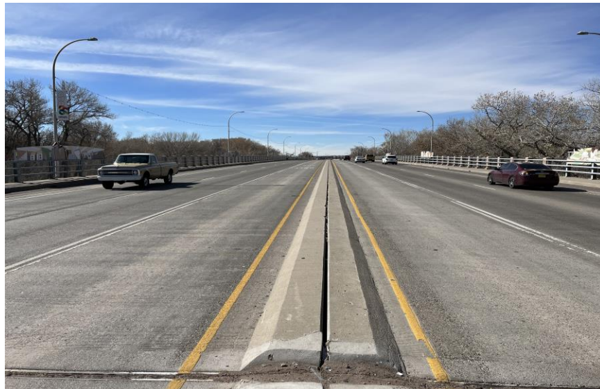
Figure 4 View of Intersecting Joint between Bridge Deck Segments
