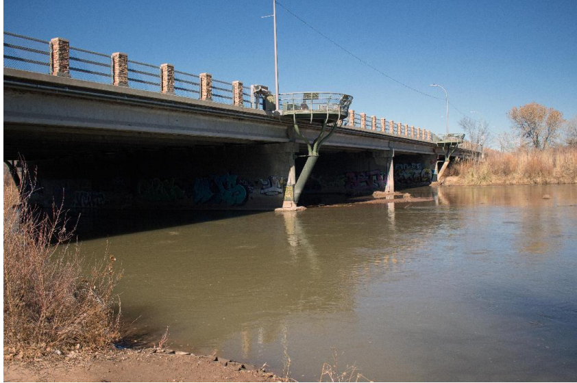
Figure 5 Photo of Rio Grande Bridge (Norman Falk Photo)
