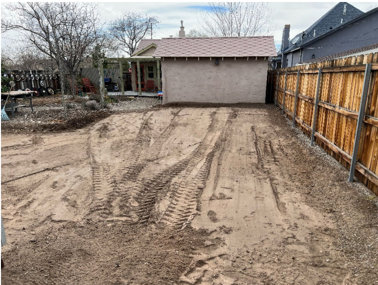
Figure 6: Subject site – view towards original garage (now a shop).
