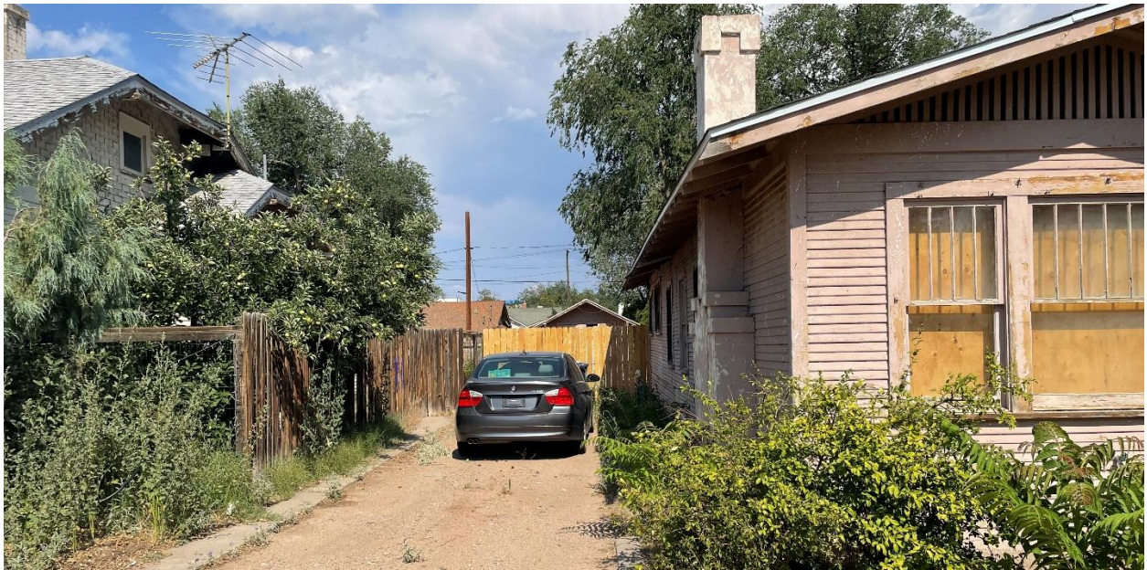
East view from 13th Street, Fence on the north side of the building
