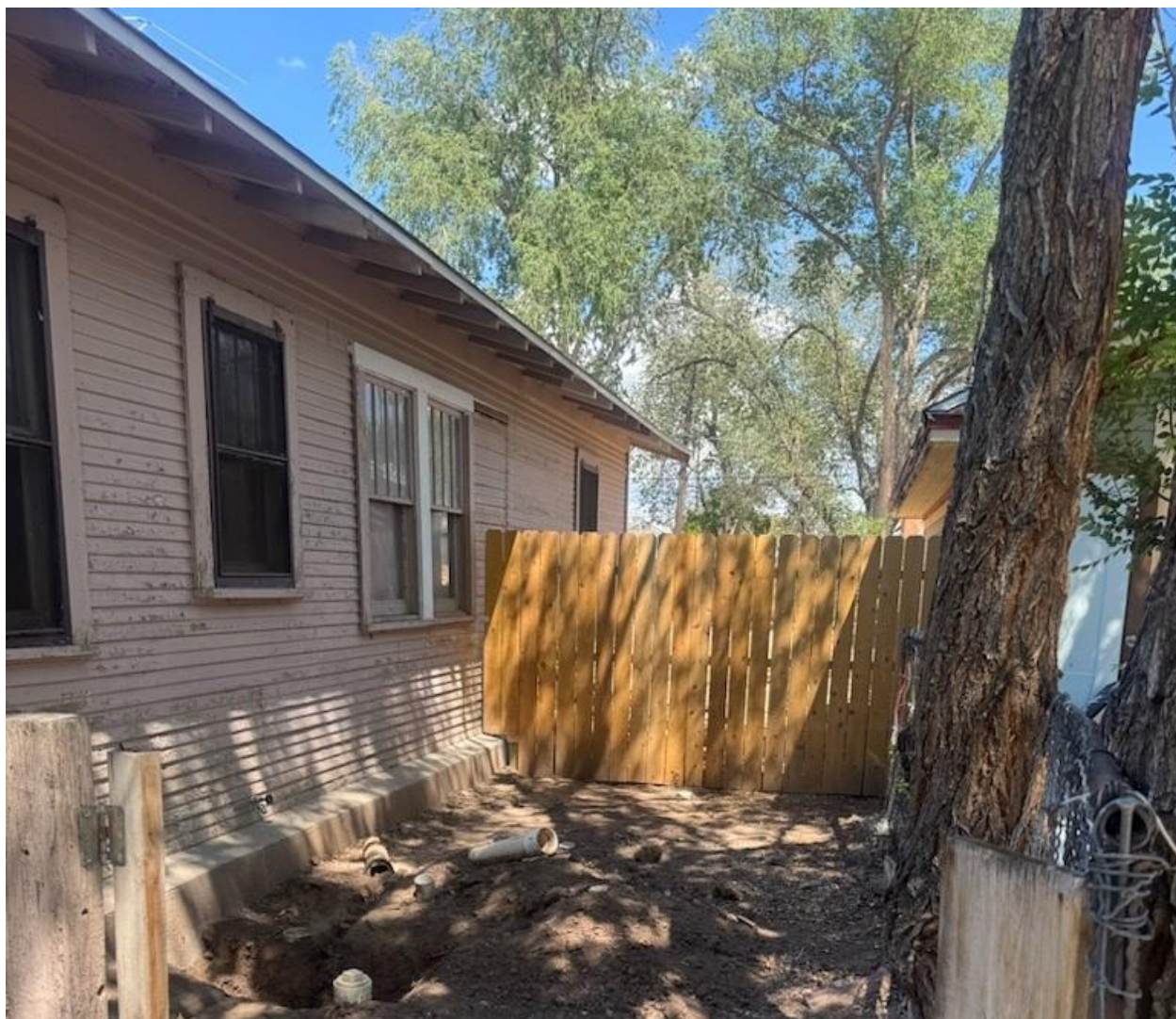
East view from 13th Street, Fence on the south side of the building
