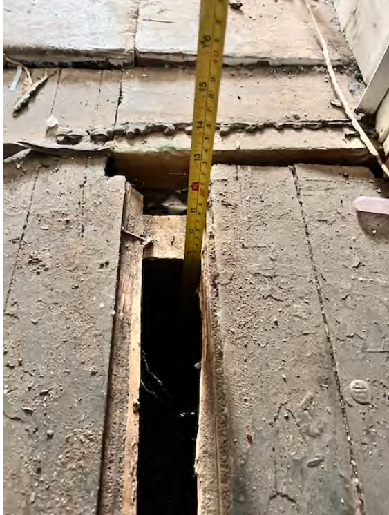
Existing floor joists sit directly on dirt
