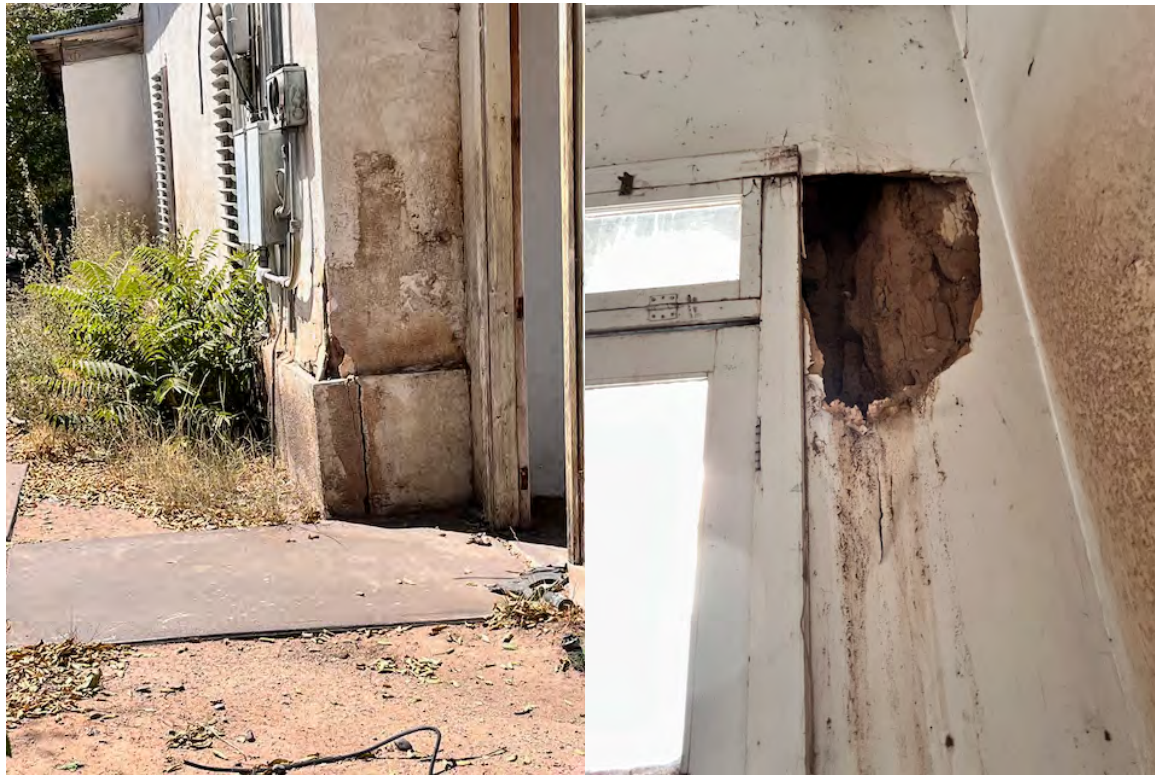
Deterioration NE corner of original structure Adobe wall deterioration at front door
