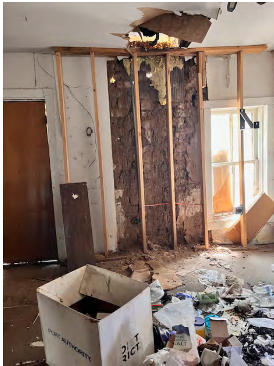
Exterior adobe addition wall collapsing
