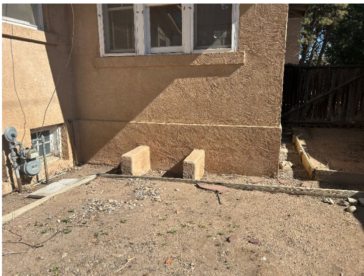
Figure 7: Perpendicular walls leading to coal chute.
