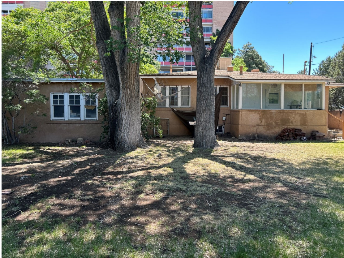
Figure 15: Rear of property.
