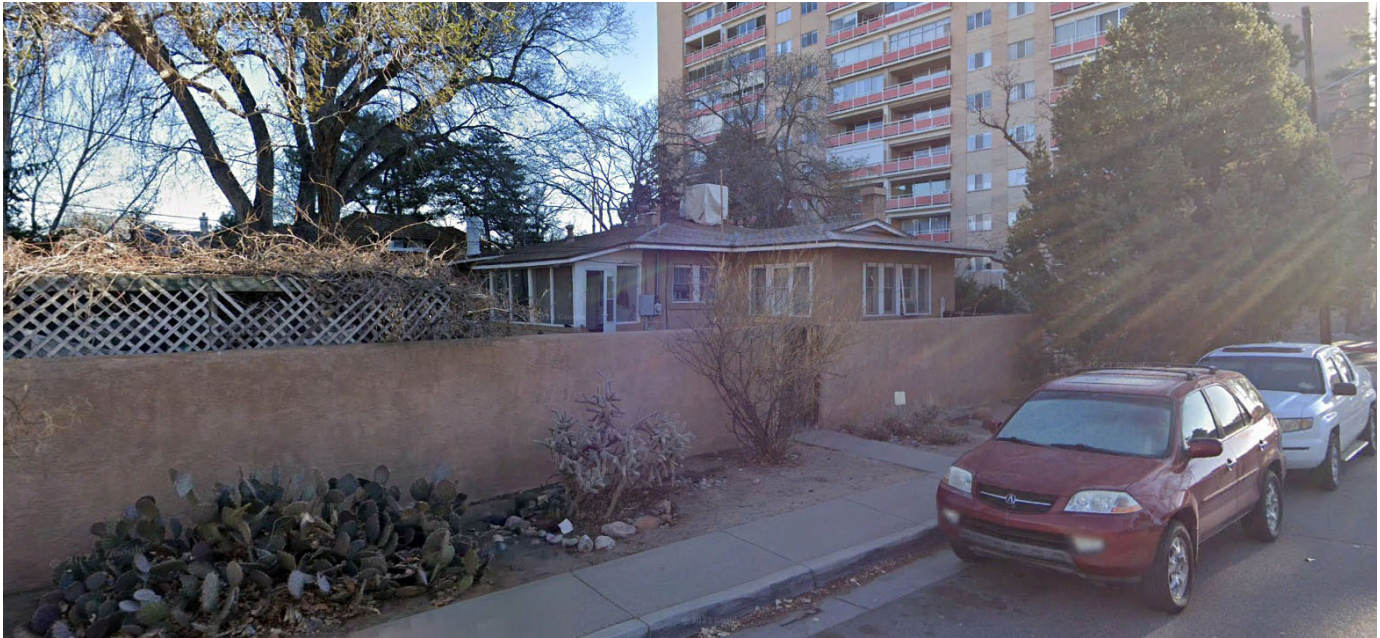
Figure 14: Street view – rear of property.
