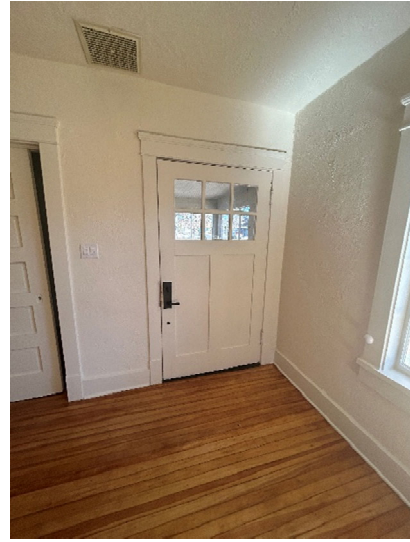
Figure 10: Original front door.
