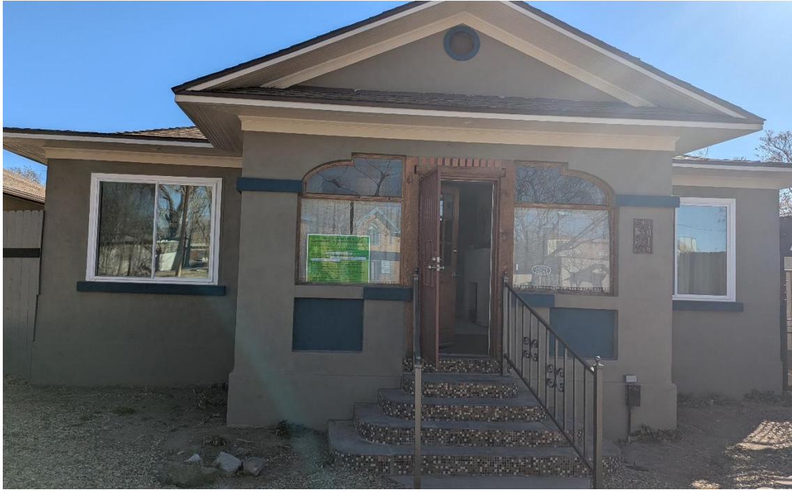
Front of the building with the Certificate of Appropriateness hearing death sign
