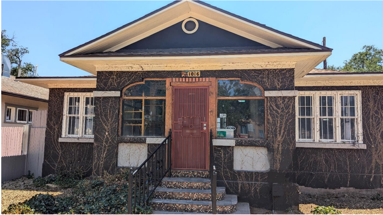
Front of the building before the renovation and changing of the original windows
