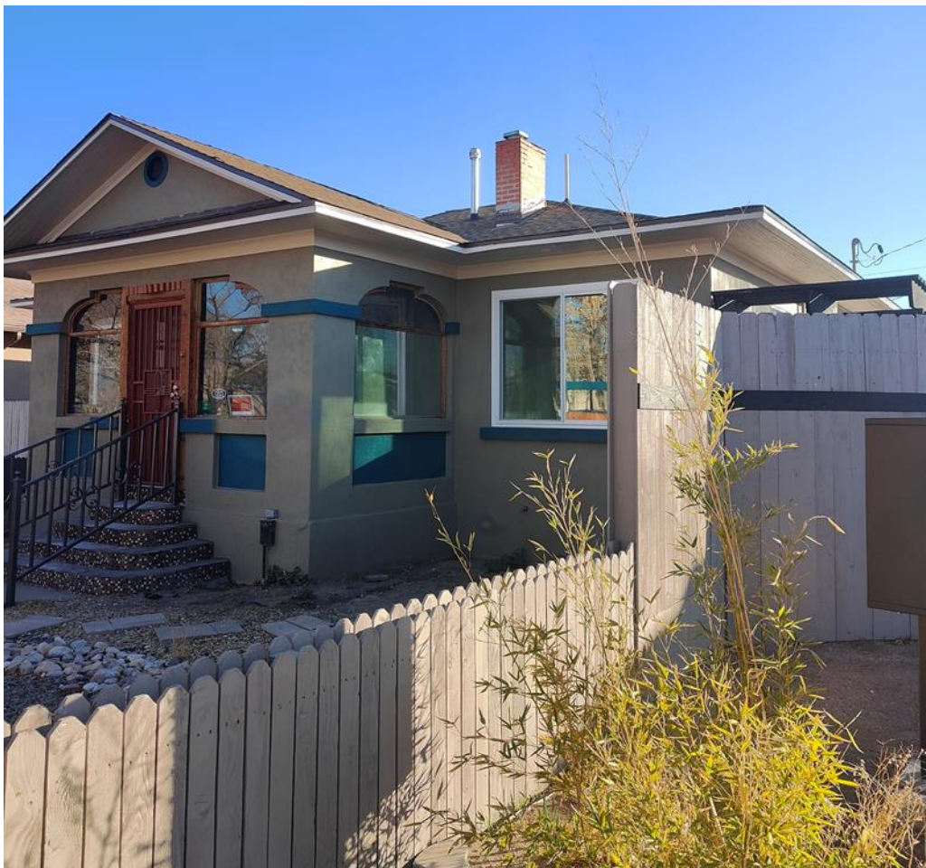
Front of the building looking Southeast.
