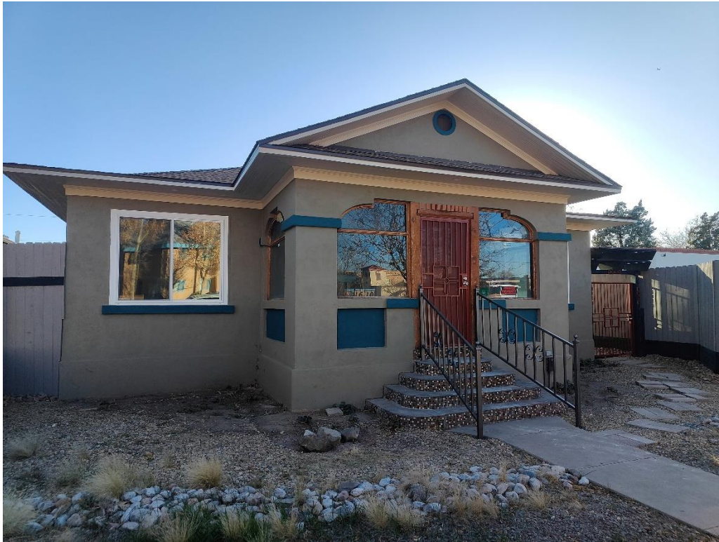
Front of the building looking Southwest.
