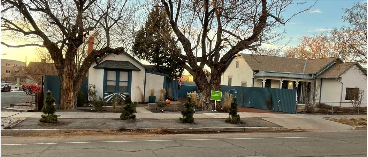
Front of the building looking west.
