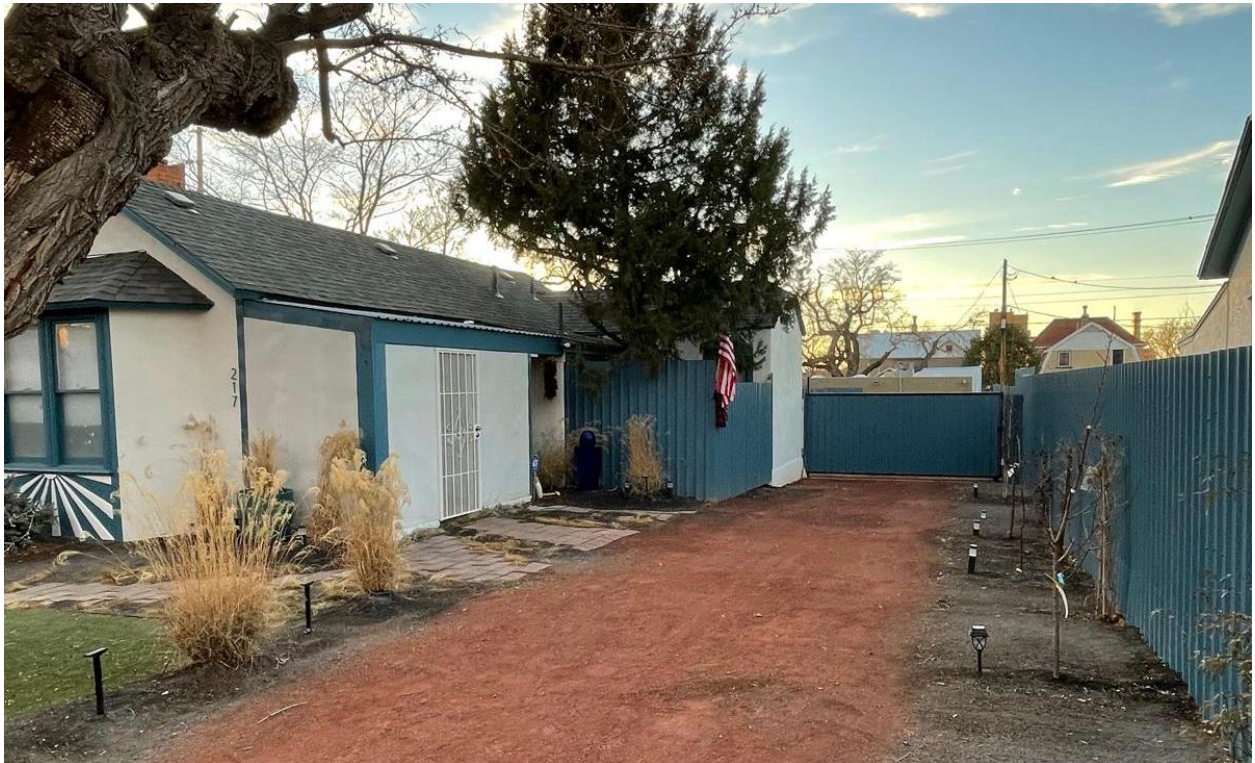
Front of the building looking west.
