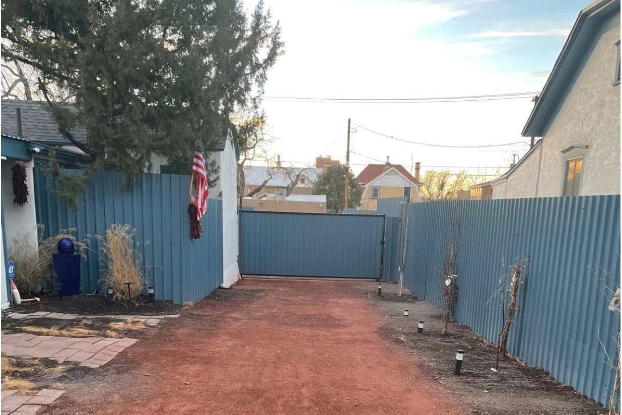
Front of the building looking west.
