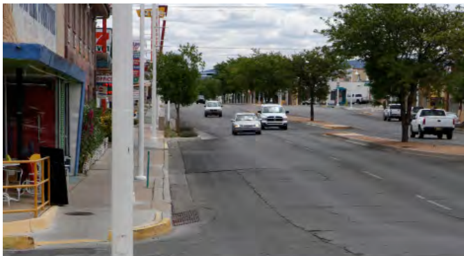
Parking lane with incomplete bulbout and no solid stripe edge.
