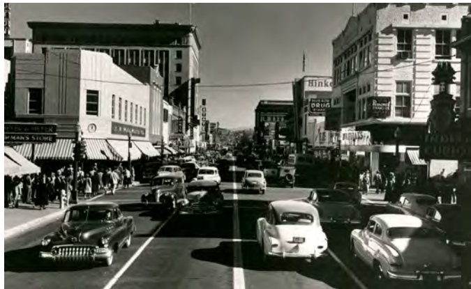
Historic Route 66 / Central Avenue(2)
