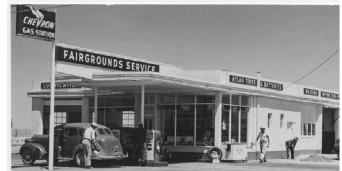
Fairgrounds service station, (1)
