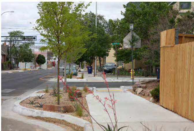
Bulbout improvement on Lead Avenue.
