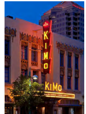
Kimo Theater Sign, Refurbished
