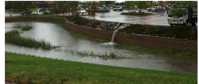
Stormwater detention.
