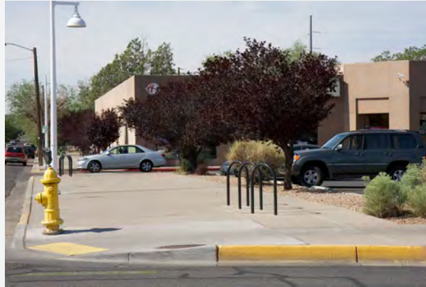
Existing area with excess sidewalk condition.
