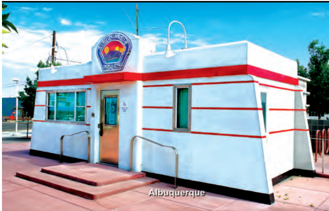
Triangle Substation, Nob Hill (1)
