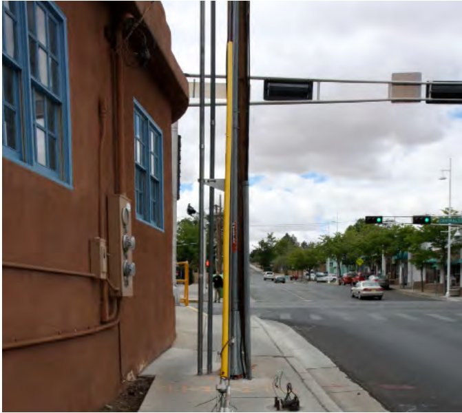
Utility poles and wires impede walking zone.
