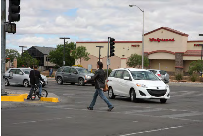
Vehicular and pedestrian conflict. Free right turn lane encourages turns against the light, threatening pedestrians in crosswalk.
