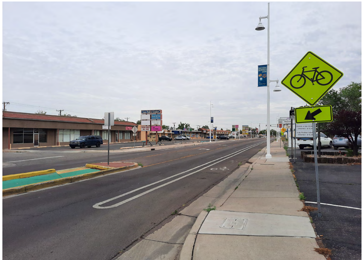
The City installed buffered bike lanes along San Pedro Drive as part of a road diet in which one lane of traffic was removed in each direction to reduce travel speeds and create safer conditions for people walking and biking.
