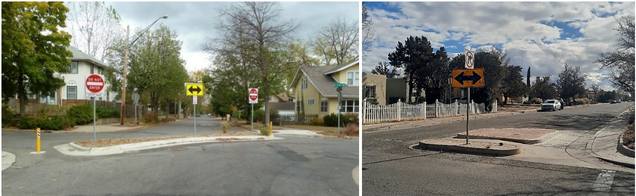
Figure 23: Example of Diagonal Diverter and Partial Street Closure with Bicycle Cut Through along Local Street
