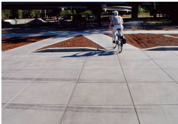
Split path entry eliminates need for bollards
