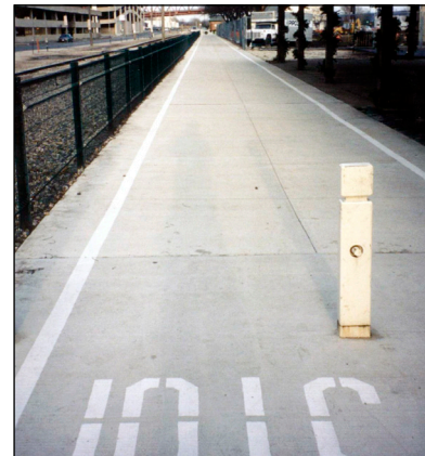
Example of swing-down bollard to allow emergency and maintenance vehicle access
