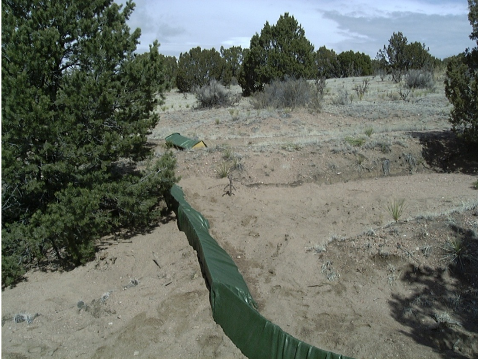
Triangular sediment filter dike
