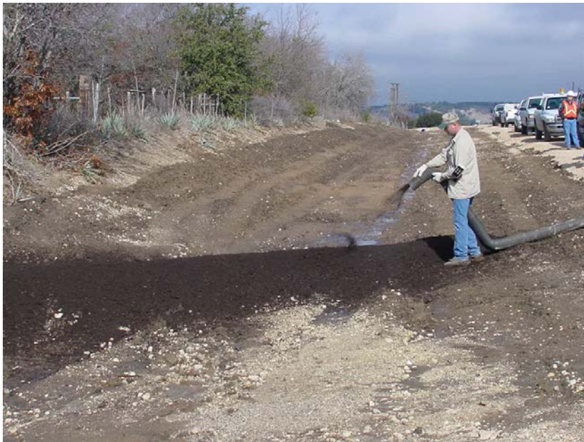
Compost berm under construction
