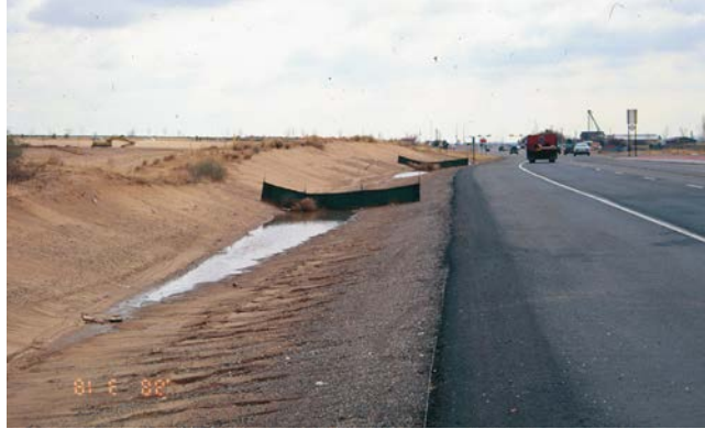
Check dams at roadside ditch
