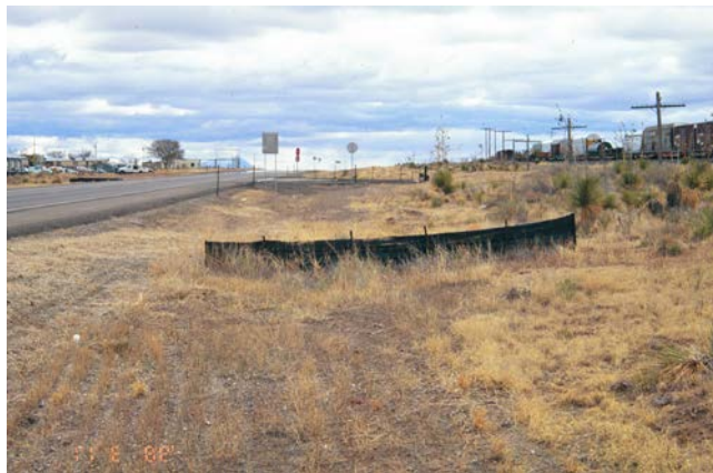
Check dam at roadside ditch
