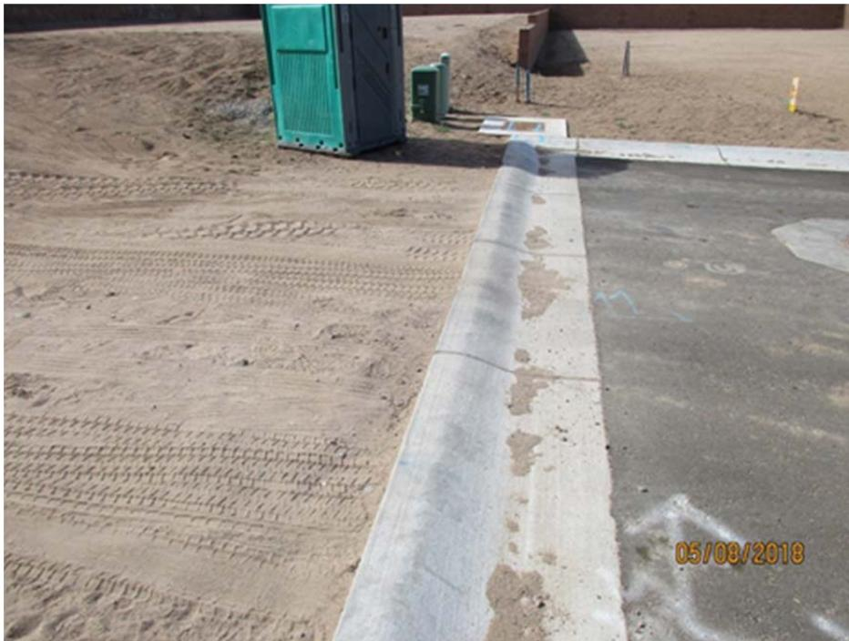
If this was the only sediment in the street, it would be acceptable. This does not mean the sediment BMP on the lot is acceptable.
