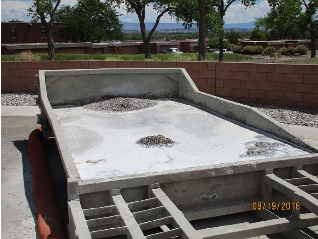
Roll-off style of wash-out facility. This container also has ramps so the pump can also be discharged into the roll-off.
