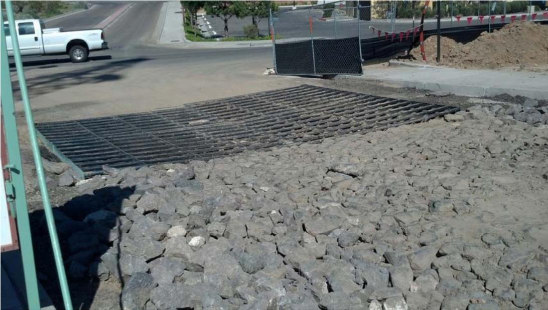
Metal grate type of Vehicle tracking control BMP with aggregate.
