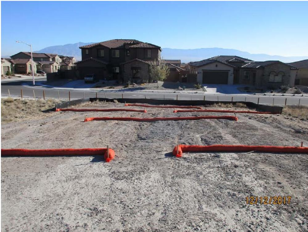
Filter socks installed on a slope to prevent erosion. This area should have been stabilized.
