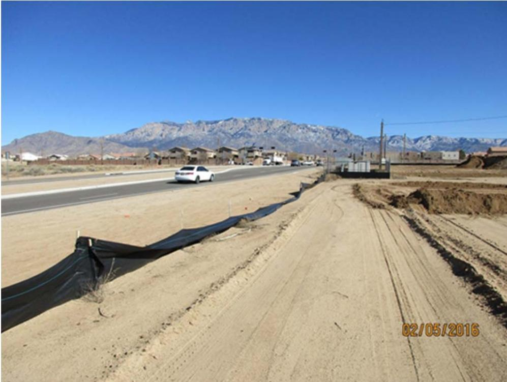
Typical result when silt fence is installed with small (3/4" x 3/4") poles spaced too far apart.
