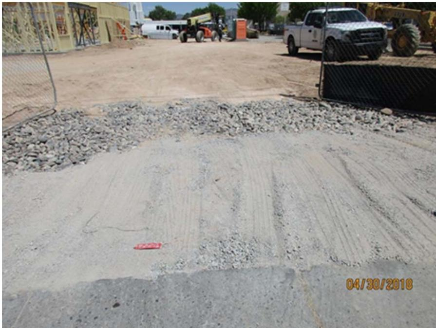
Track-out pad is too short. In addition, fine material was tracking-out onto the street.
