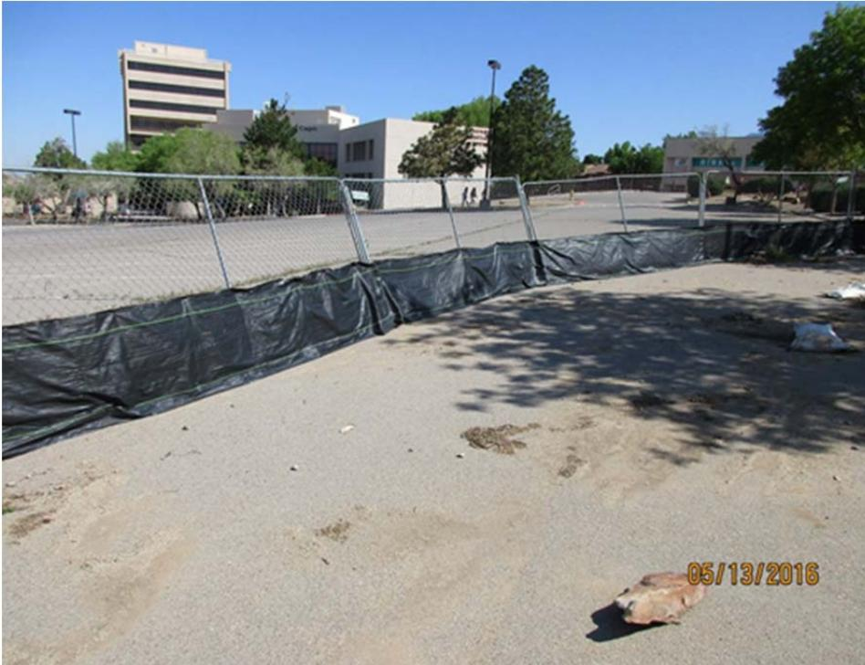
Silt fence installed across an impervious surface.
