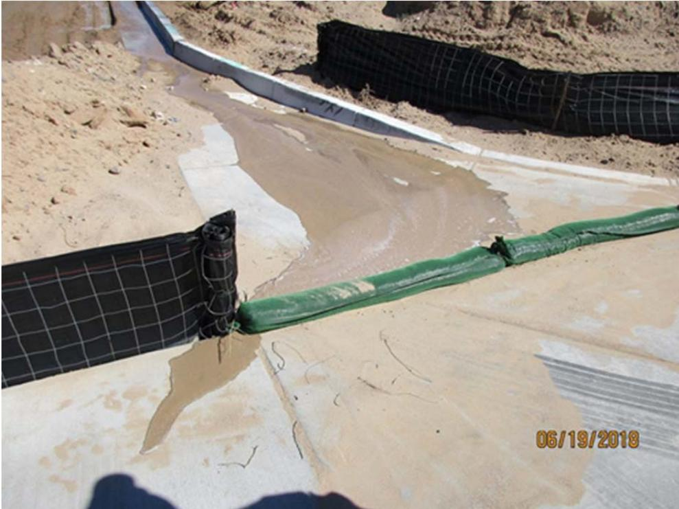
Flow under rock sock at joint. If it was turned uphill and overlapped the silt fence, it may not have leaked.
