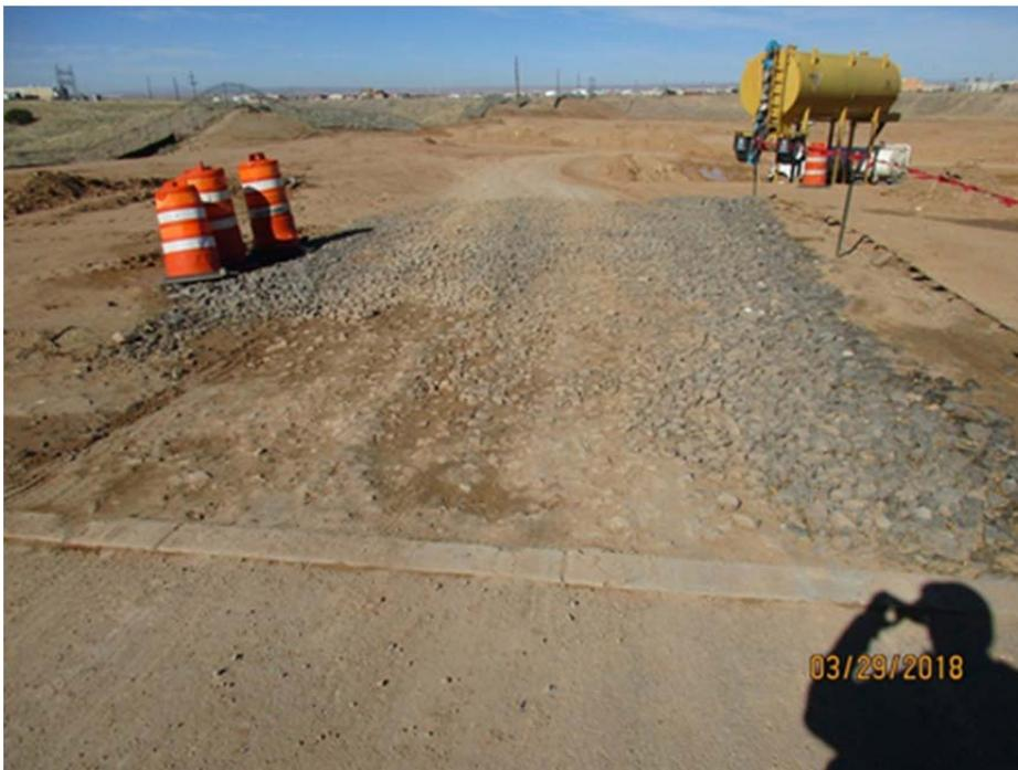
Track-out pad requires maintenance. Not enough aggregate is available for track-out control. Replenish or replace aggregate as it becomes clogged with sediment.
