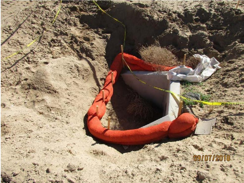
Open storm drains are considered an inlet and require protection. This also includes storm drains that are not actively being worked on.
