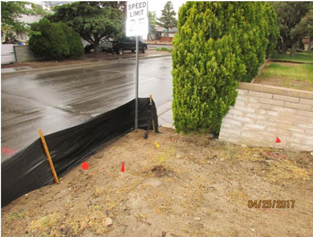
Gap in silt fence. Silt fence should have been extended to the block wall. This corner is a drainage outfall for the site.
