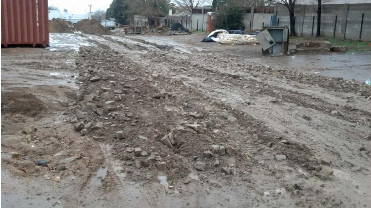
Example of a muddy site, wherein, vehicles shall not be entering the roadway except to leave the job site for the day. The contractor at this project shut down receiving dirt trucks for the day.
