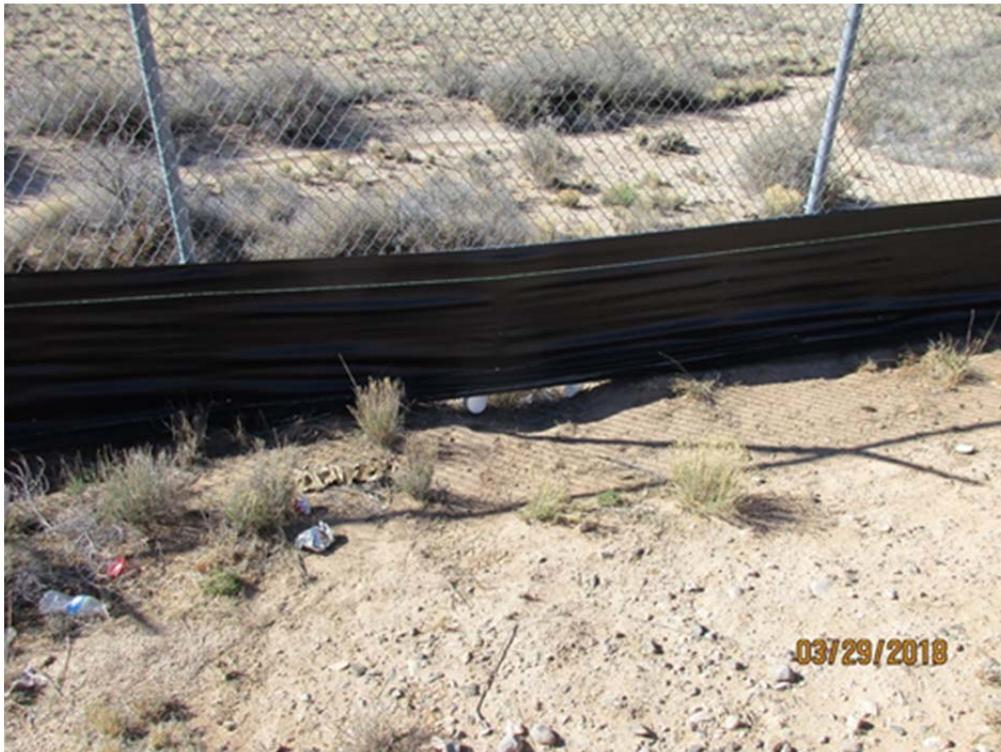
Gap between silt fence and the ground. Sometimes placing a mulch sock in this location is the easiest way to mitigate this condition.
