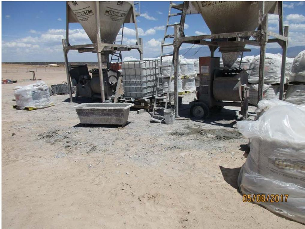
Mortar towers with plastic beneath as a BMP.
