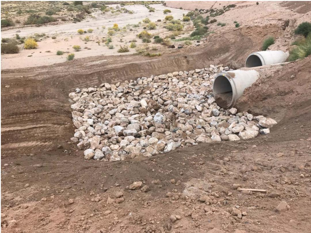
Energy dissipator for large storm drains
