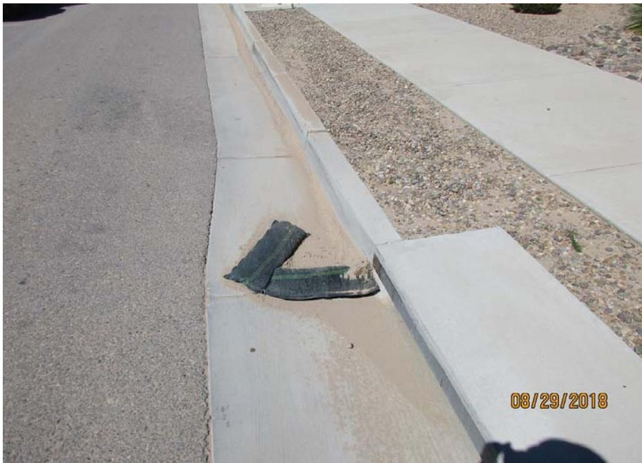
Inlet protection requires maintenance since sediment is to the top of one rock bag and the bags no longer form a "T".
