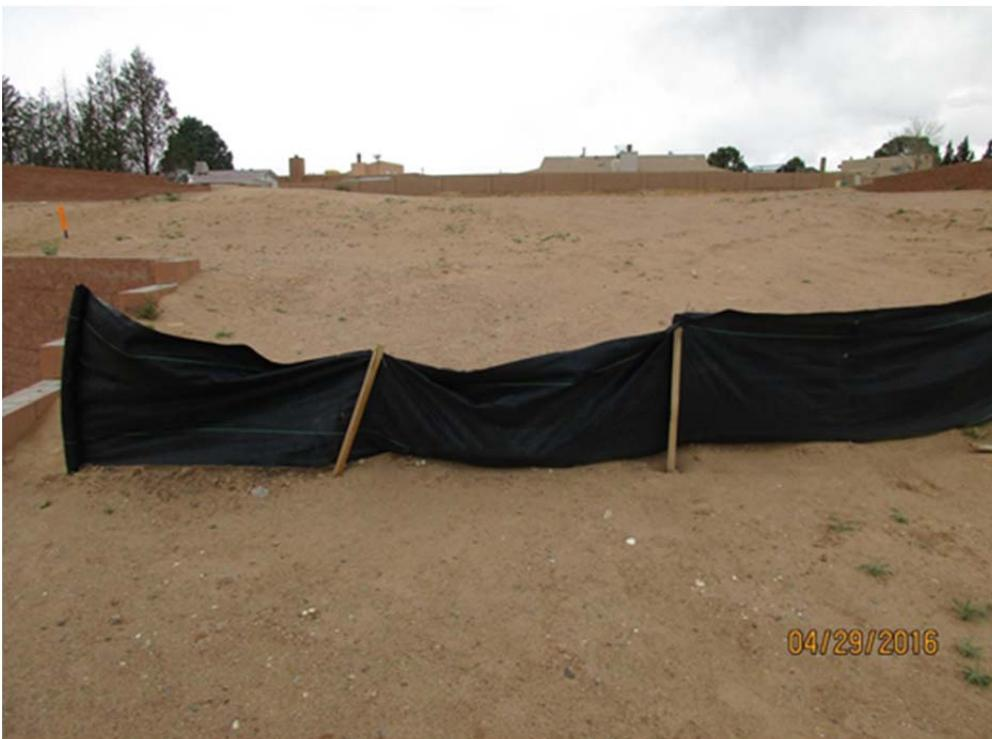
Silt fence installed with  $\frac{3}{4}$ " x  $\frac{3}{4}$ " poles that are not strong and these poles were not adequately buried.
