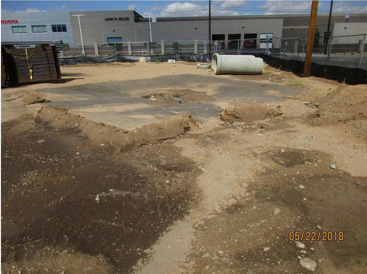
Uncompacted berm got “Blown-out” during a storm.
