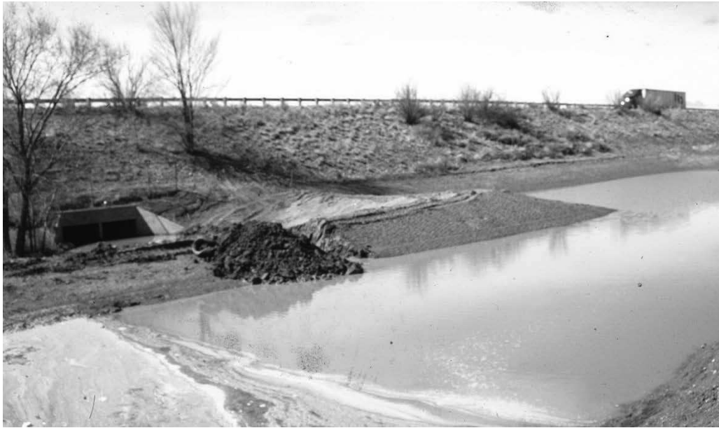
Sediment pond at inlet of box
