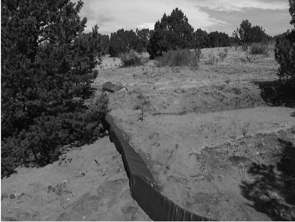
Triangular sediment filter dike
