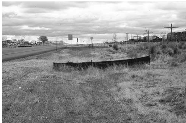
Check dam at roadside ditch
