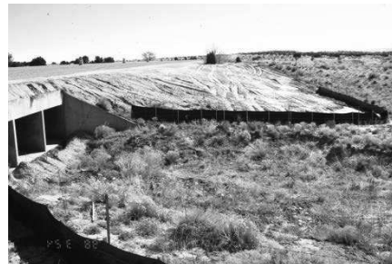
Silt fence at outlet of box
