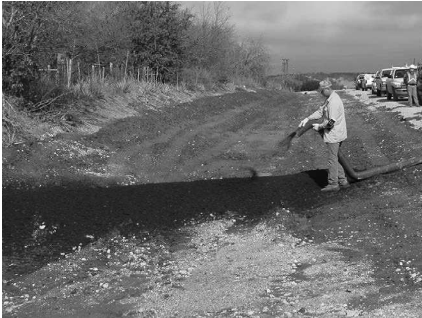
Compost berm under construction
