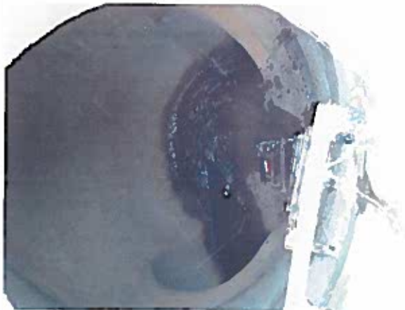
A small amount of flow observed in the Outfall D2 manhole.
