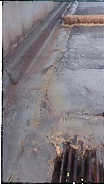
Storm water flow into Outfall PY1.
