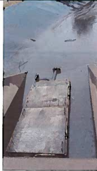
Sheen observed at Outfall PY3 sample location.
