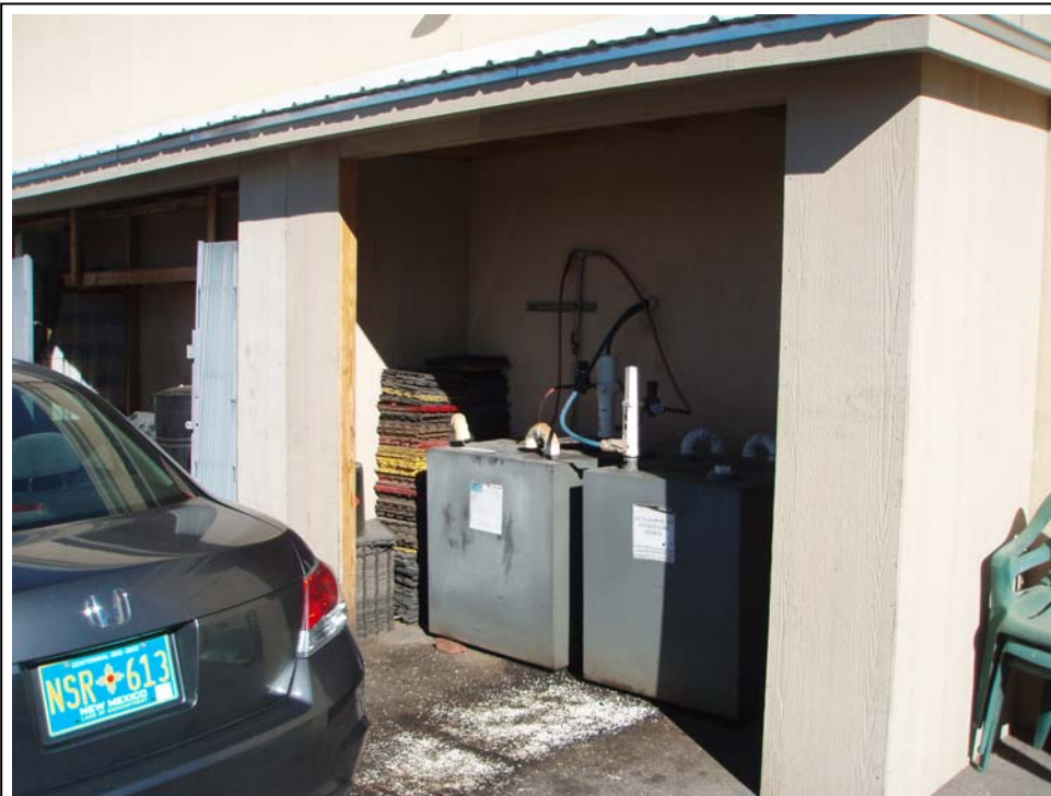
4. Example of outdoor storage tanks that are in good condition and under cover, but with staining still visible from oil transfers
