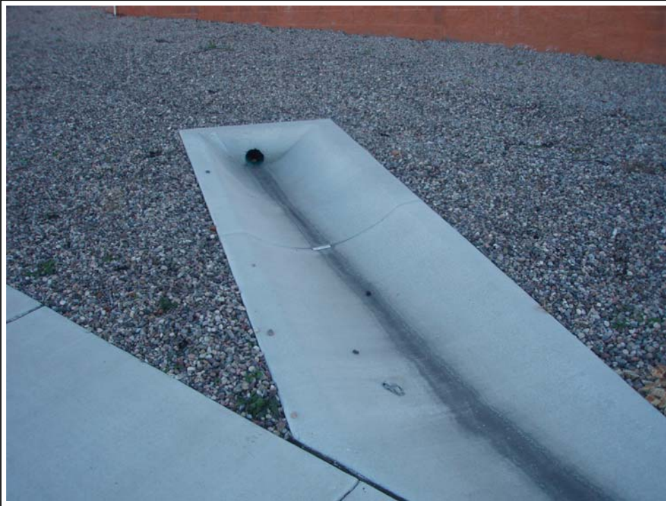
1. Staining at a drain that connects to storm drain system
