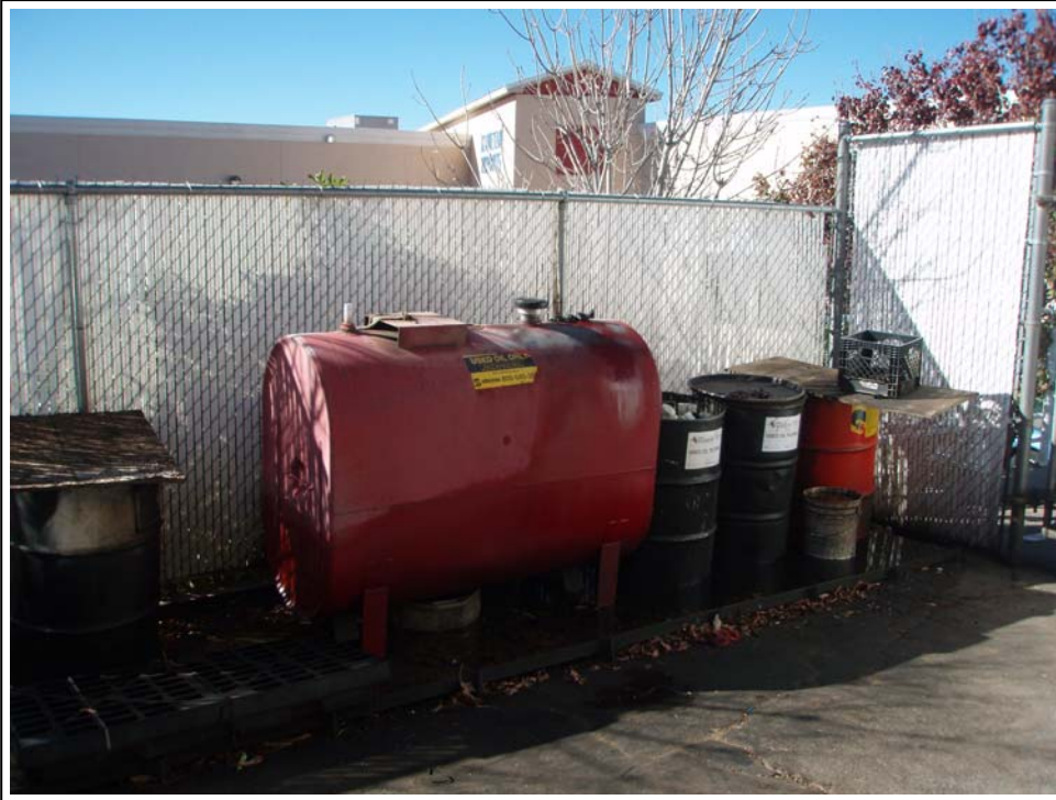
3. Example of business using some BMPs, with room for improvement by covering drums and adding pumping secondary containment
