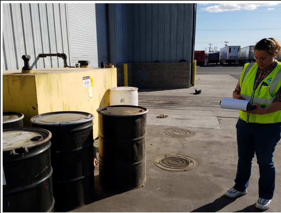
2. Example of outdoor storage: covered drums and tank in good condition but no secondary containment
