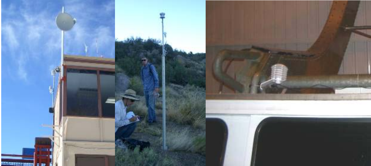
Figure 1-13 The locations of HOB0 temperature/relative humidity sensors at the roof of the Sandia Tramway building at the peak (left), at the base of the Sandia tramway (middle) and on the roof of a tramway car (right)
