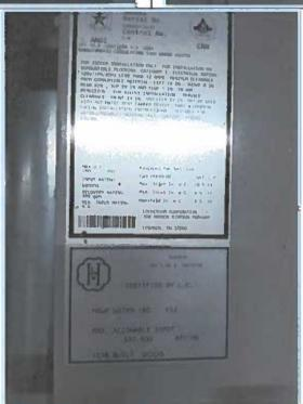
Emission Source: Domestic Water Boiler #2 LOCHINAV CORPORATION Model No. CWN500PM Serial Number C05H00175132 Input Rating 500,000 Btu/hr
