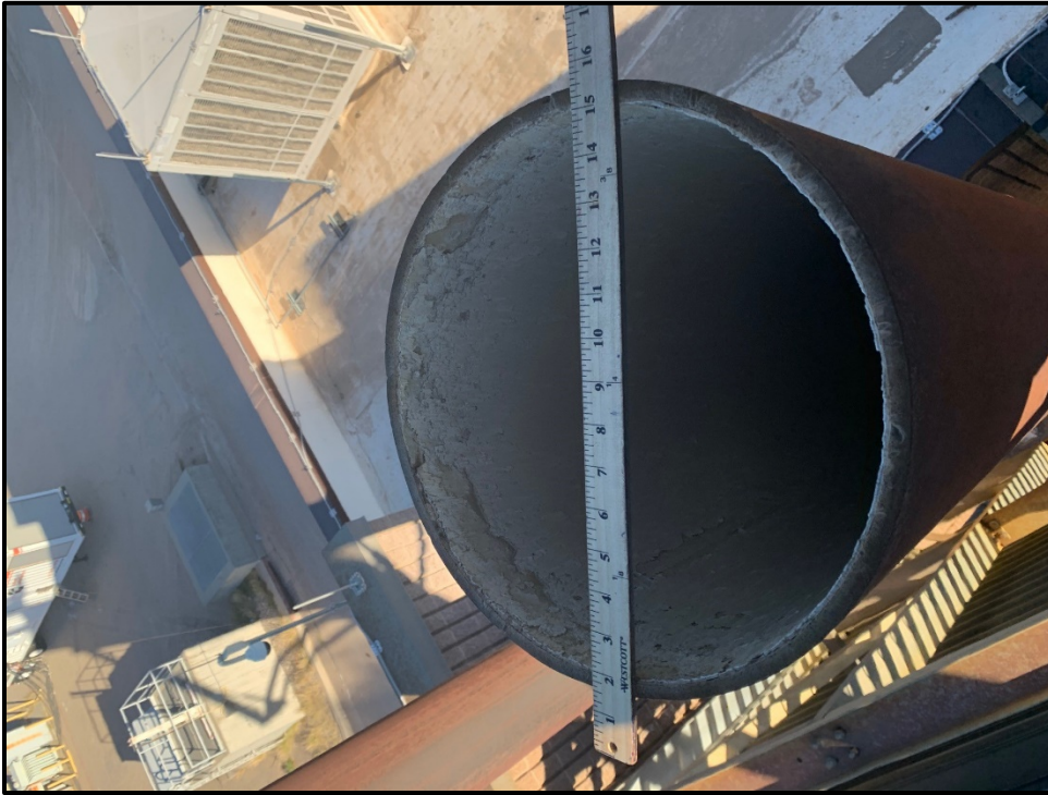
Figure 11: EU: 29 Stack Diameter Measurement
