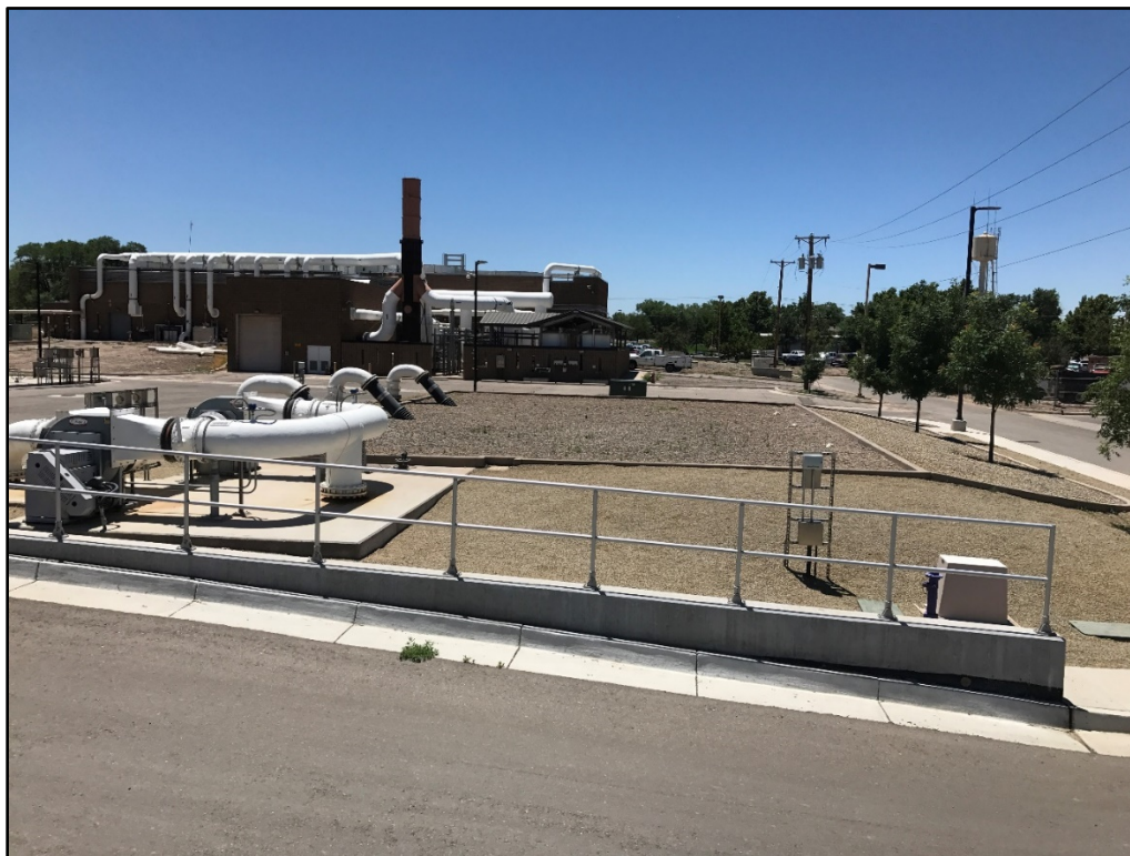
Figure 2: Picture of a Bohn Biofilter
