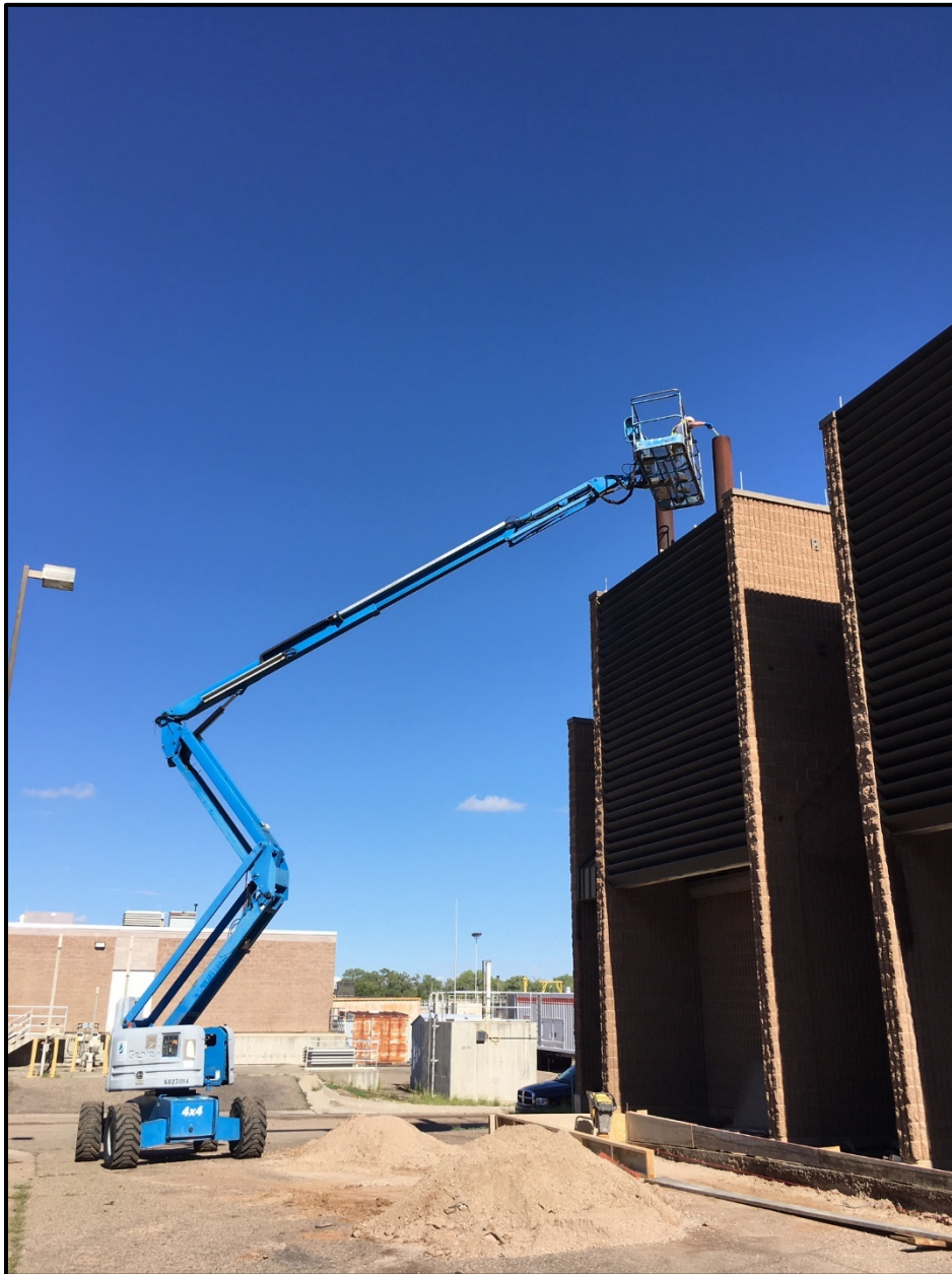
Figure 8: Field Measurements Taken to Confirm Cogenerator Stack Parameters
