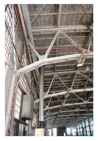
Blacksmith Shop, Steel Truss at column surrounded by masonry wall.
