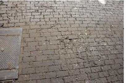
Machine Shop Floor, 3" thick Kreolite creosoted woods blocks sit on a 6" thick concrete floor to dampen sound
