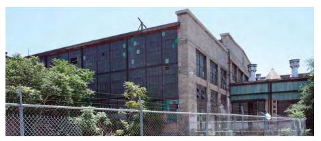
Northeast corner, Reinforced concrete with fully glazed perimeter wall.
