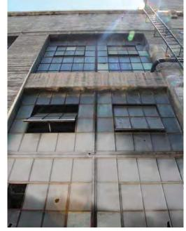
West elevation, Glazing inset to concrete frame.
