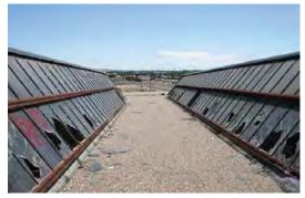
Built-up roofing, positive slope to South.
