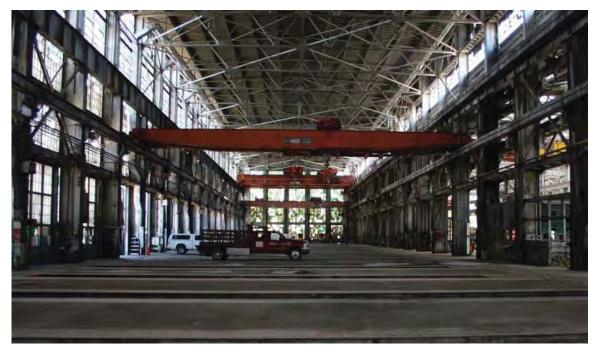
Machine Shop, Erecting Bay, 57' clear height to underside of truss structure. Floor troughs can be seen across slab.
