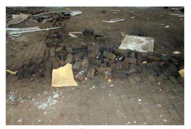
Damaged flooring, 3" thick creosoted end-grain wood blocks
