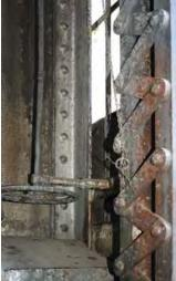
Crank mechanism for skylight operation.
