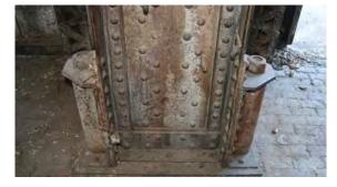
Erecting Bay columns supported on deep piles, dampened by springs.
