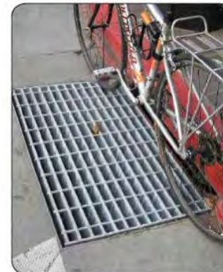
Examples of bicycle-safe drainage grates.
