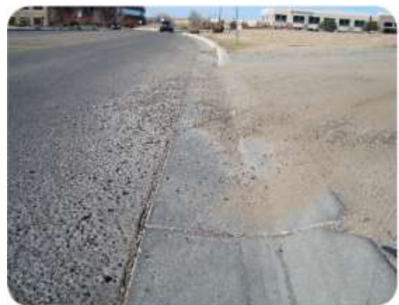
Figure 71: Unwanted Gravel and Sand on a Bike Route from Unpaved Driveway
