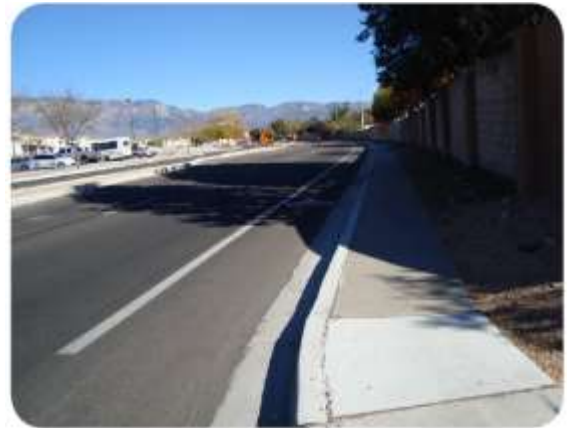
Figure 69: Pavement Overlay with Smooth Gutter Transition
