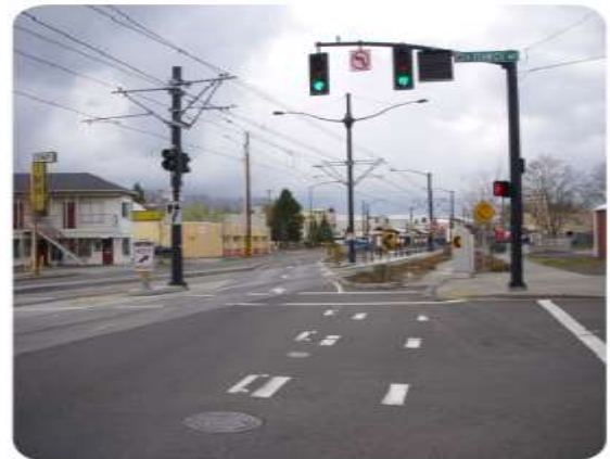
Bike lane dashed through complex intersection.
