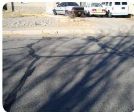
Figure 68: Crack Sealed Pavement
