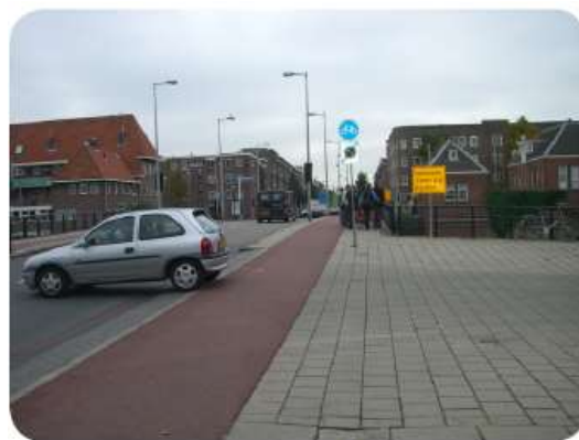
Cycle tracks should be continued through driveway crossings, improving visibility.
