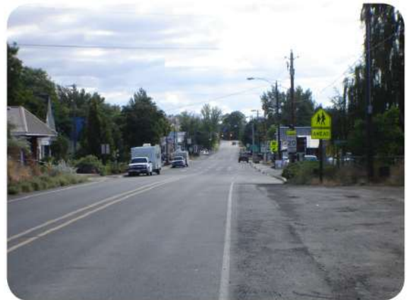
Roadway widening is preferred on roads lacking curbs, gutters and sidewalks.
