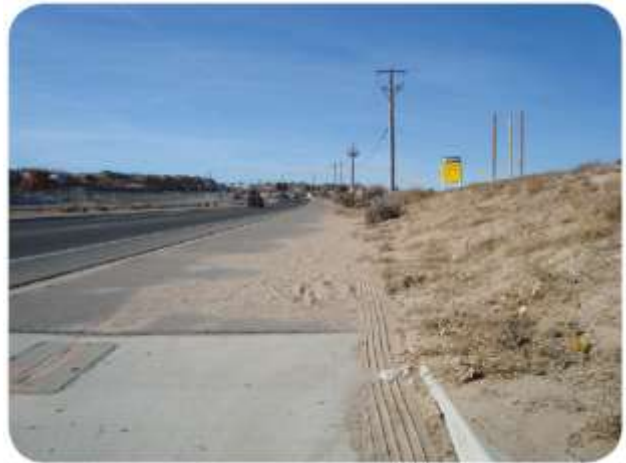
Figure 79: Sand from Storm Runoff Deposited on Multi-Use Trail
