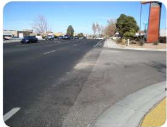
Figure 73: Debris from Storm Water Runoff
