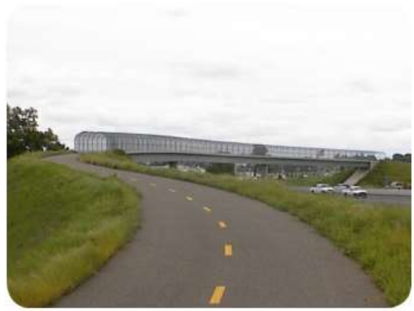
Type 4 Grade-Separated Overcrossing.
