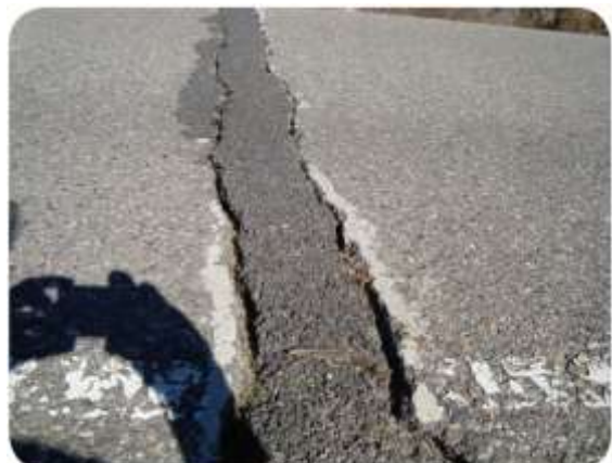
Figure 74: Pavement Crack Repair Using Rigid Material, Pulling Away from
