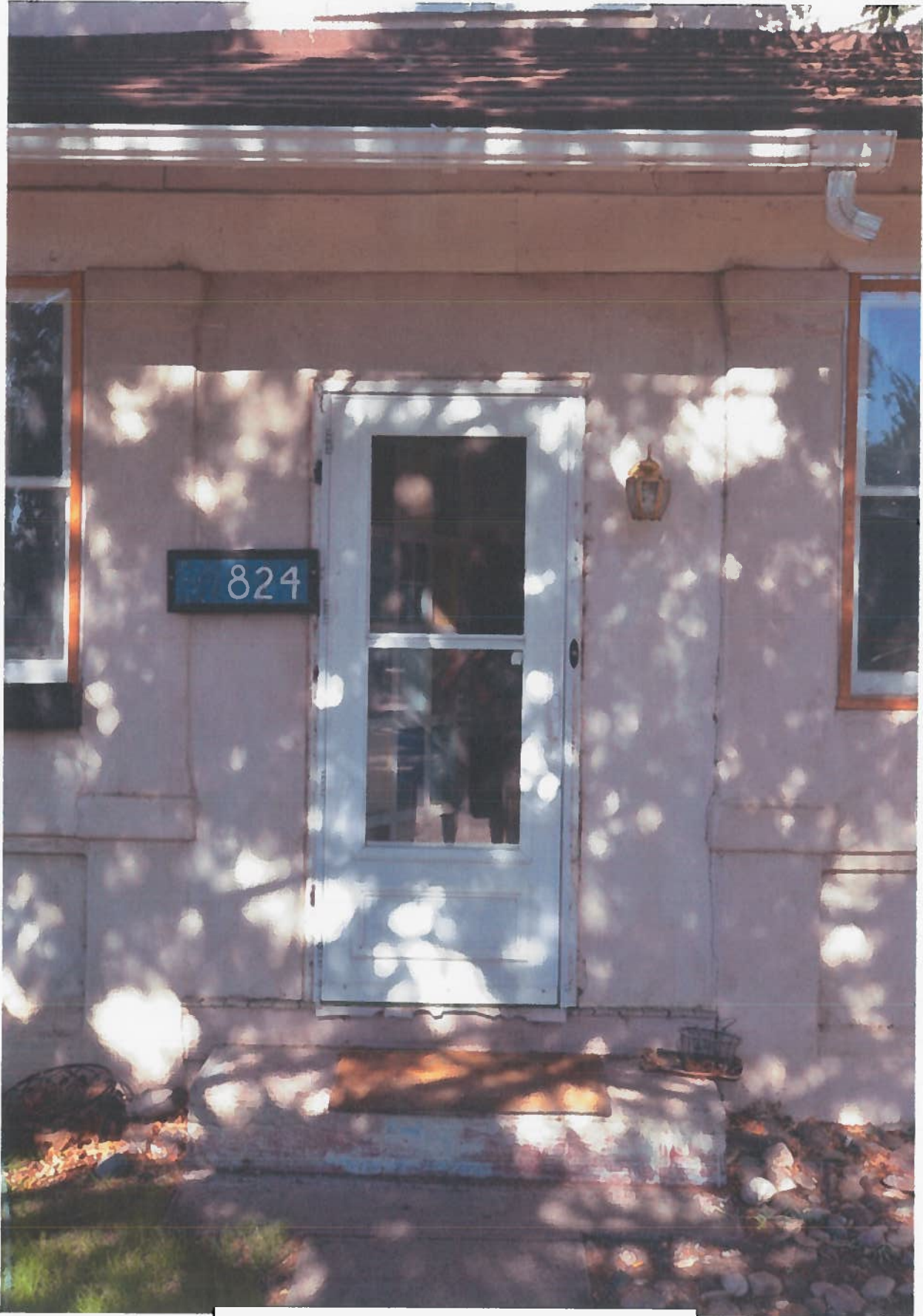
Attachment A-1 Existing Pilasters at Front Door
