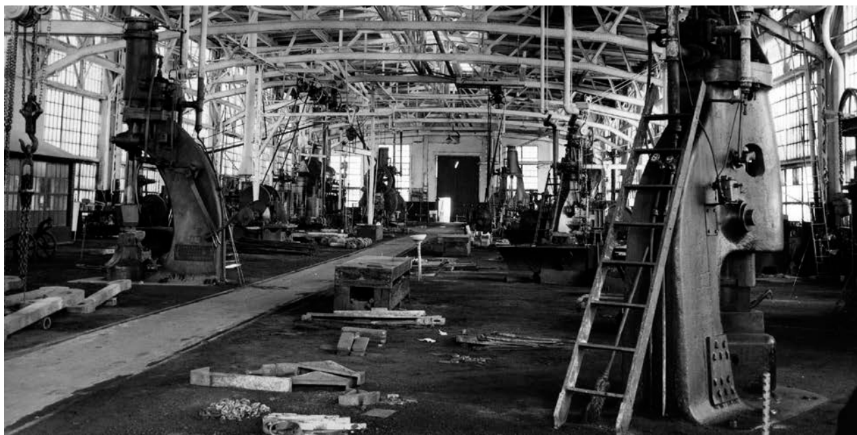
Figure 7. View of blacksmith shop interior with presses. Steel trusses span the full width of the blacksmith shop.
