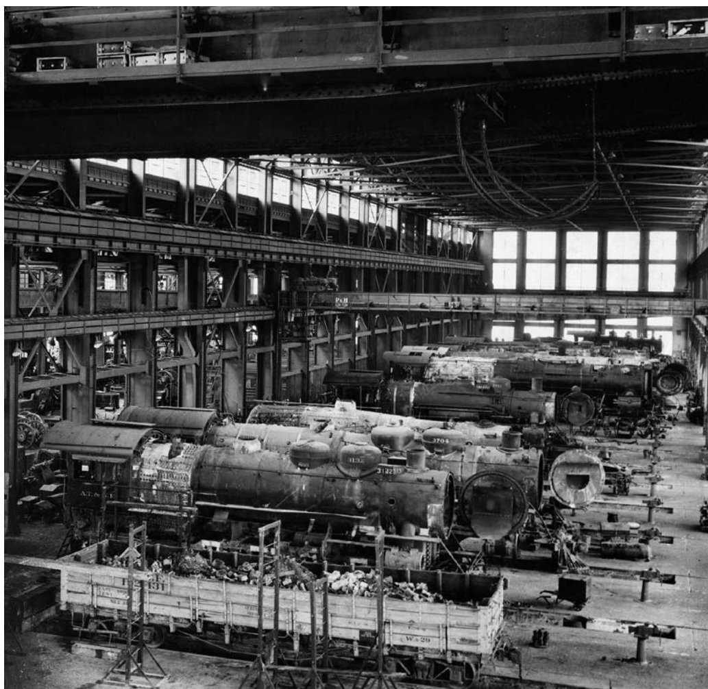
Figure 3. Locomotives in the erecting bay, looking southwest, note concrete pits and 250 ton bridge crane above.
