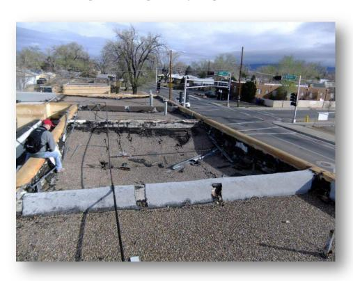
Figure 18- Building C Partially Collapsed Roof Structure
