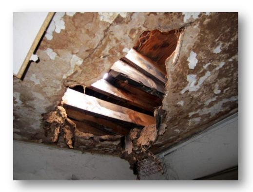
Figure 7- Building A Room 106 - Ceiling Collapse - Exposed Structure
