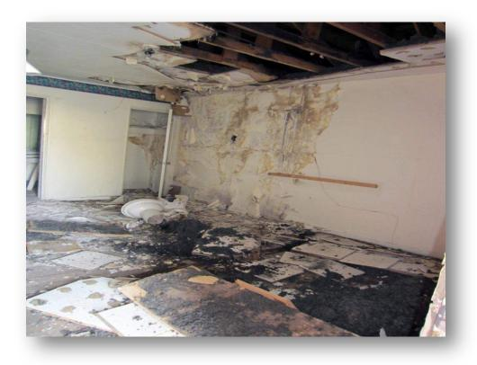
Figure 2- Building A Room 102 Ceiling Collapse
