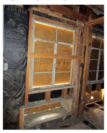
Figure 15- Building B Room 110 - Cut Exterior Studs
