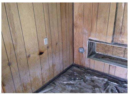
Guest Room Side Wall Heating/Cooling Unit Receptacle With Surface Mount J-Box
