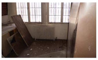
**Figure 2 - Typical Steam Radiator with Manual Control**Page 3
