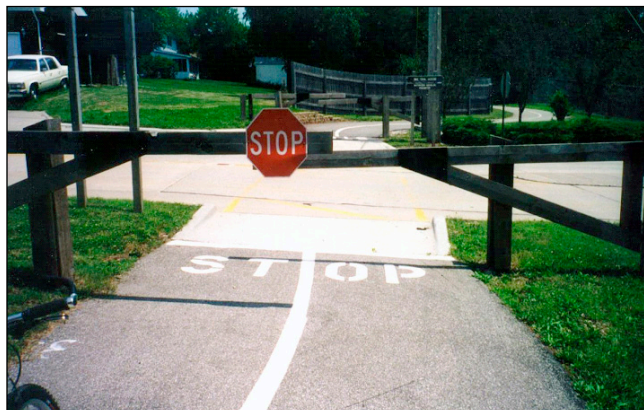
Figure 5-21: Gates across a bicycle path (not recommended)
