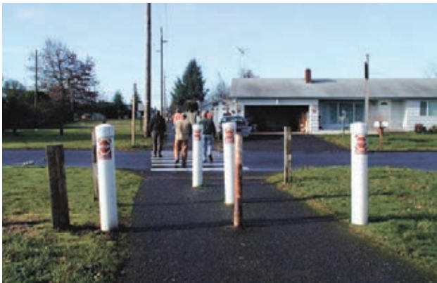
Bollards are overused and can cause injury
