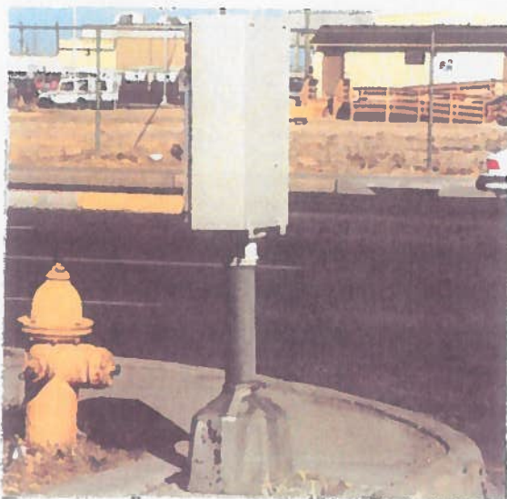
On the left, a traffic controller blocks the sidewalk probably because of the proximity of the adjacent fire hydrant. With no curb ramp, getting on the sidewalk would be difficult anyway. On the right, a crosswalk leads a pedestrian to an island with no curb ramps.
