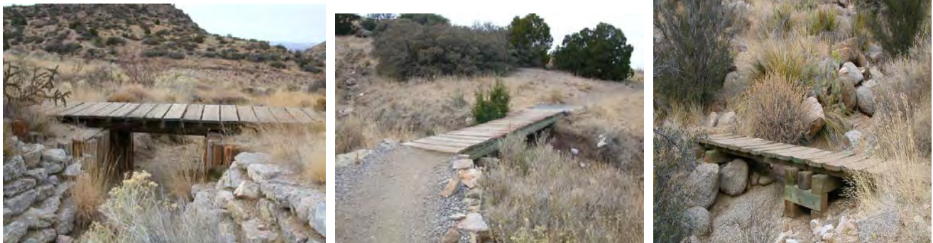
Various structures made from natural wood and rock materials help bridge drainages.
