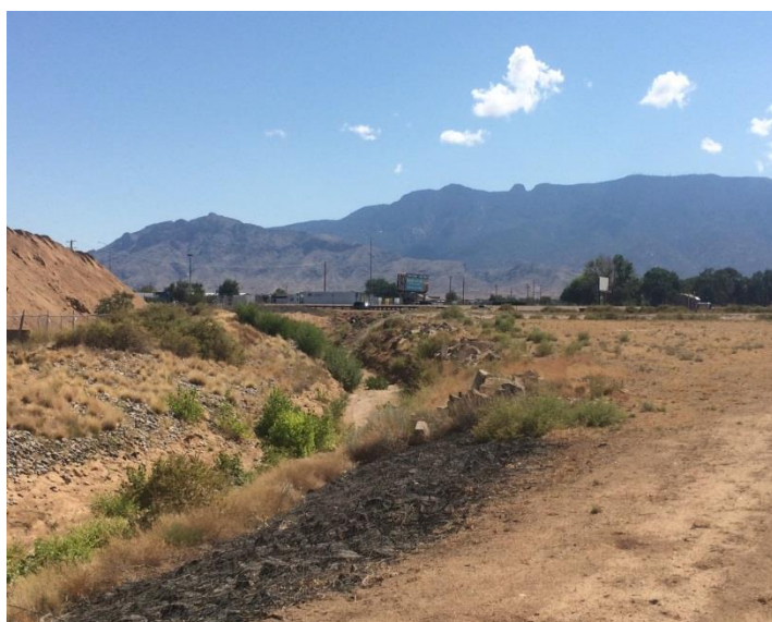
Figure 6 –Deteriorating drainage channel
