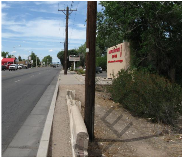
FIGURE 4-7 Unpaved and Obstructed Sidewalk
