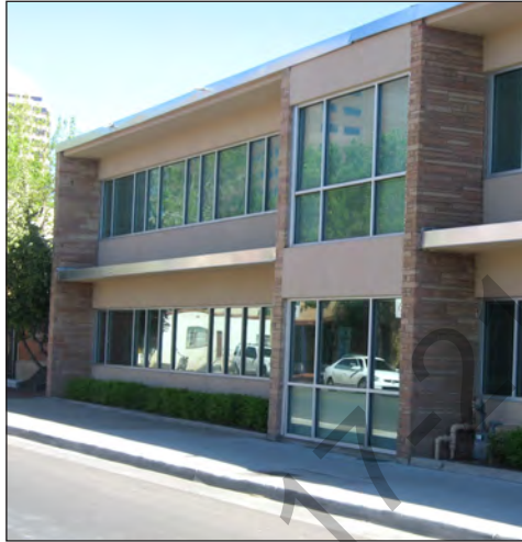
Office Building on Eighth St. - windows cover more than 50% of the ground floor façade and 30% of the second floor façade.
