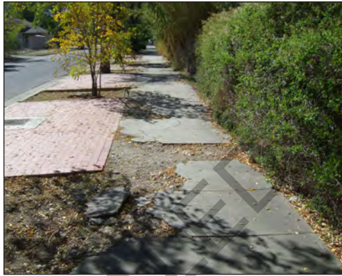
Deteriorated sidewalk
