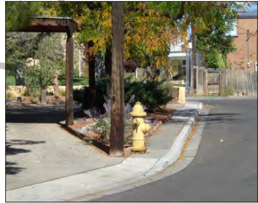
Fire hydrant obstructing very narrow sidewalk
