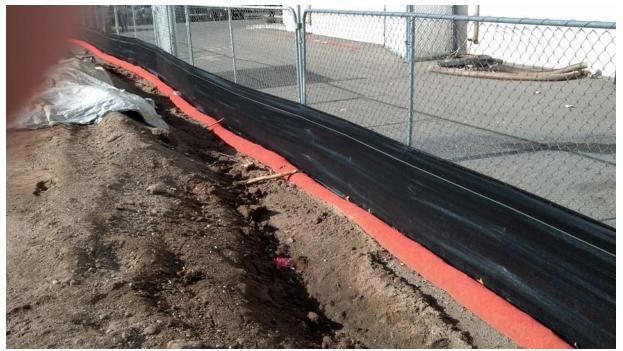
Mulch sock installed at bottom of silt fence to "seal" on an impervious surface.
