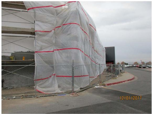
Plastic sheathing used to contain Styrofoam during rasping.
