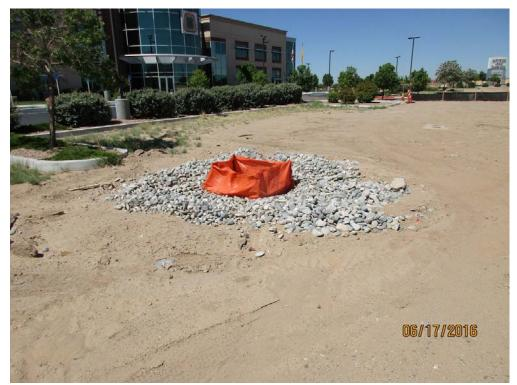
Silt fence style of inlet protection. This Operator also used large aggregate to reduce the velocity of the flow.
