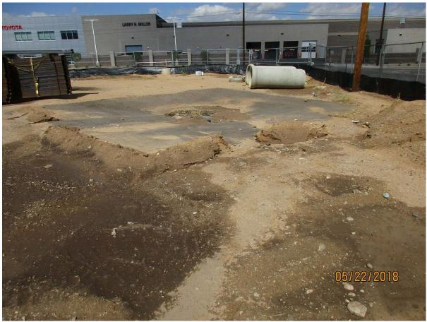
Uncompacted berm got "Blown-out" during a storm.
