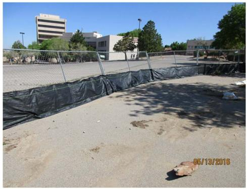
Silt fence installed across an impervious surface.
