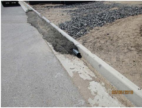
Cold-mix asphalt ramp used for accessing the site.
