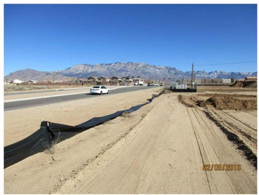
Typical result when silt fence is installed with small  $(3/4" \times 3/4")$  poles spaced too far apart.
