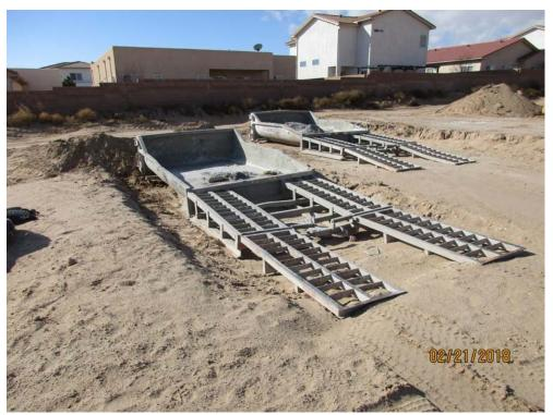
These roll-off wash-out containers were lowered for easier access.
