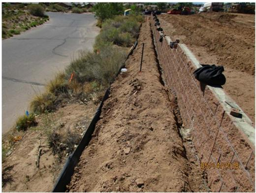
Silt fence is too full. Dirt is to be removed from behind the fence.
