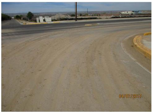
This amount of track-out was rated as heavy. Heavy track-out is thicker, covers most of the roadway and extends further from the site than medium track-out.
