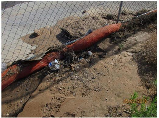
Flow undercutting beneath the filter sock. Sock was not staked down.
