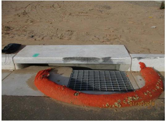
Filter sock is protecting the grate, but not the throat of the inlet. Basically it is not working.
