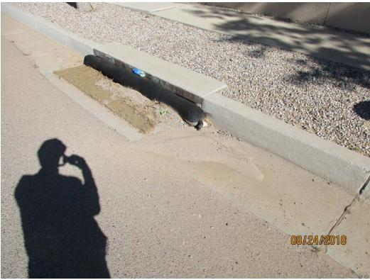
Cocoa mat grate cover with mulch sock covering the throat. It is working, but the Operator was informed it required maintenance due to the amount of sediment on the mat and upstream of the BMP.
