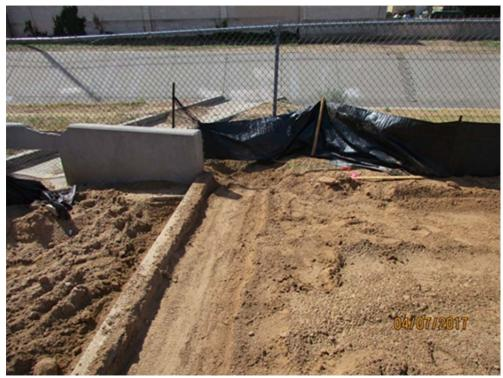
Silt fence installation with numerous issues: not buried, poles are not strong enough, fence is not taught and it is not buried. Reinstallation of this silt fence or installation of another sediment BMP is required.
