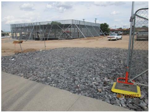
Aggregate track-out pad. Note construction fence to prevent bypass.
