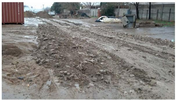
Example of a muddy site, wherein, vehicles shall not be entering the roadway except to leave the job site for the day. The contractor at this project shut down receiving dirt trucks for the day.
