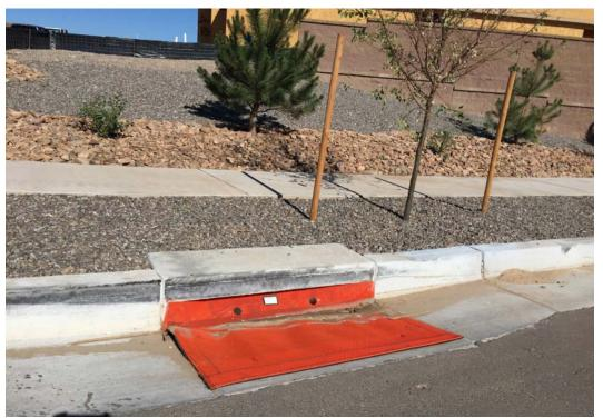
One-piece inlet protection BMP for an inlet with a grate and a throat.
