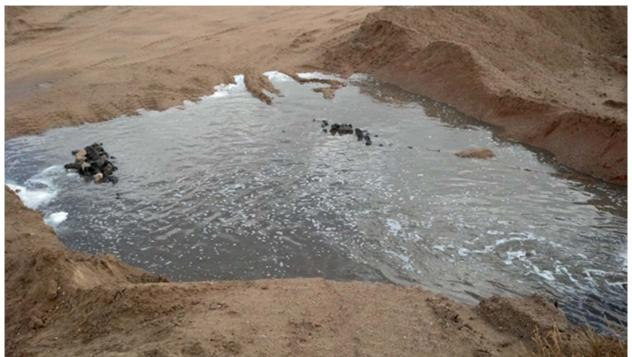
Energy dissipation (plunge pool) for slowing the velocity of water entering the arroyo under construction. This one could have used more aggregate, but it was still functional.
