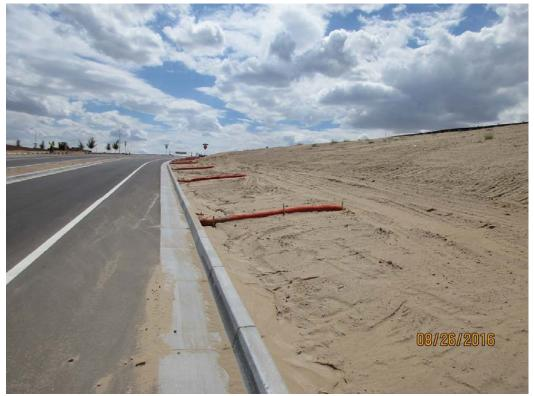
Mulch socks installed to catch sediment draining downhill behind the curb and to reduce the velocity of the water. This area should have been stabilized.
