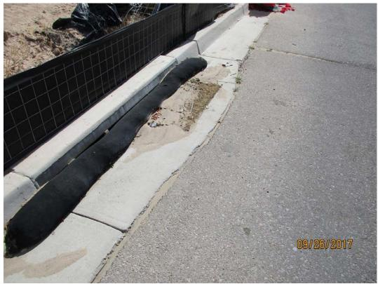
Inlet protection requires maintenance since grate is more than half-full of sediment.
