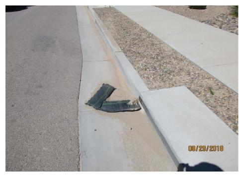
Inlet protection requires maintenance since sediment is to the top of one rock bag and the bags no longer form a "T".
