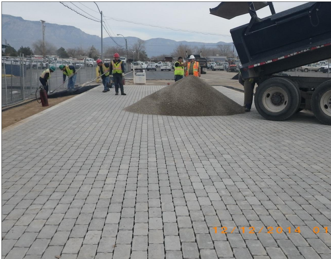
December 12, 2014, Void Filling for Permeable Pavers
