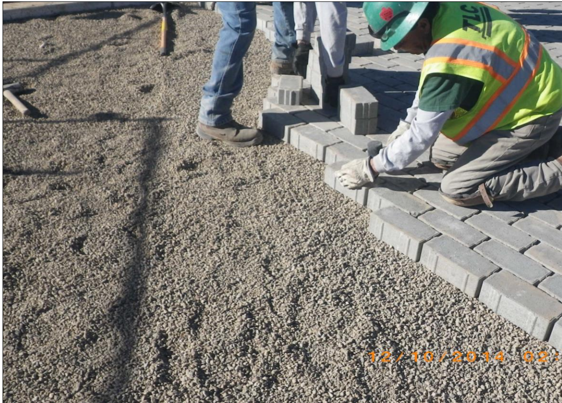
December 10, 2014, Installation of Permeable Pavers (west area)
