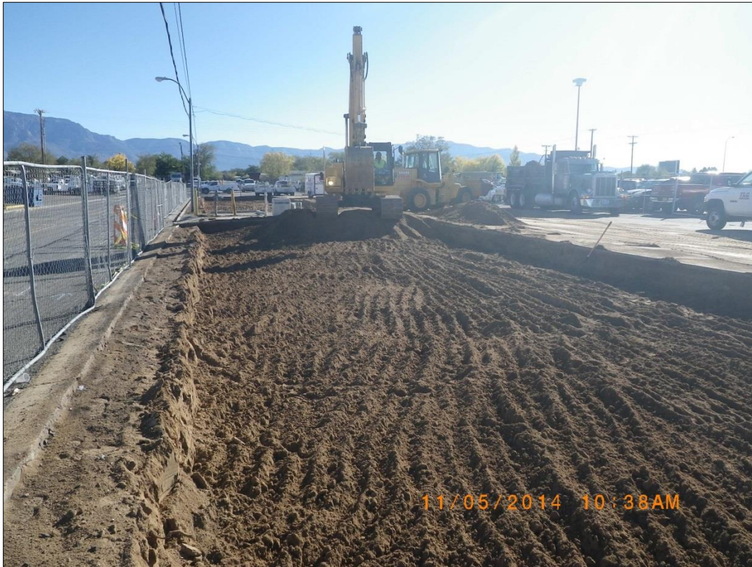
November 5, 2014, Pavement Removal and Initial Excavation
