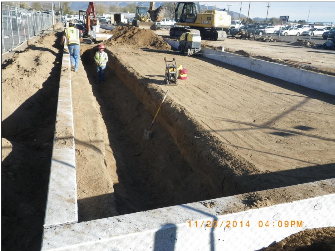
November 20, 2014, Excavation for Storage (maximum depth 6 feet)
