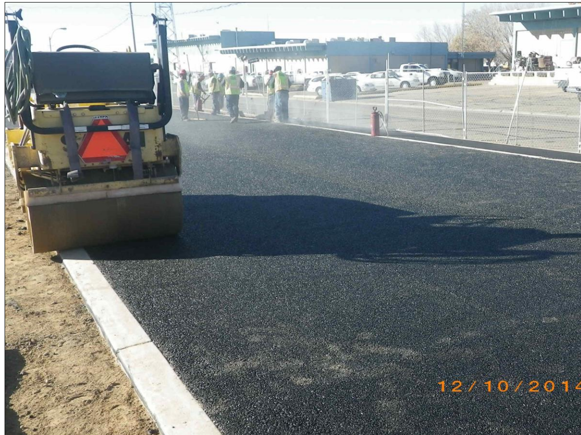
December 10, 2014, Paving with Porous Asphalt (east area)
