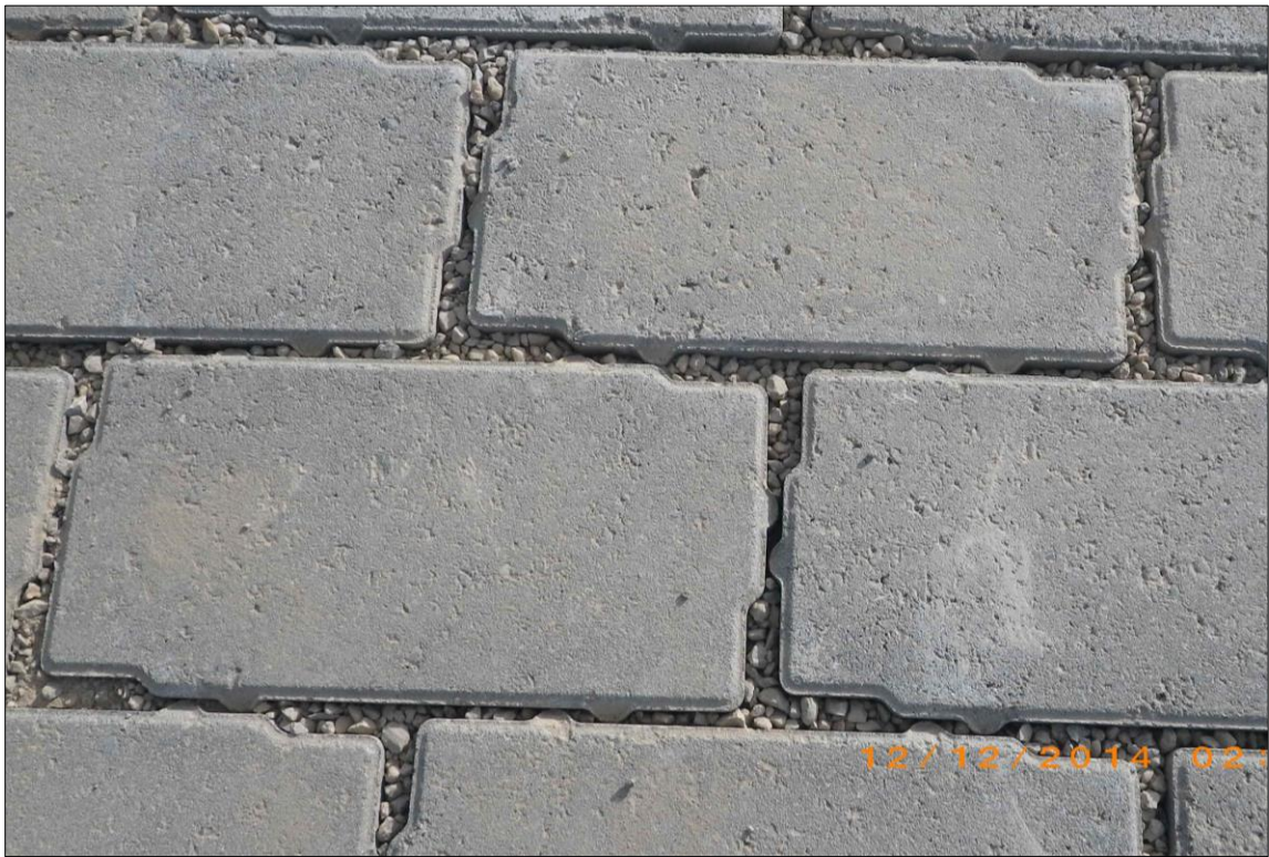
December 12, 2014, Permeable Pavers in Place
