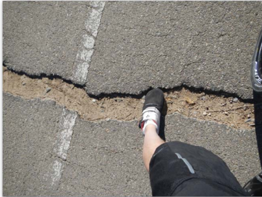
Figure 40. Segment 8, Wide transverse cracks in trail
