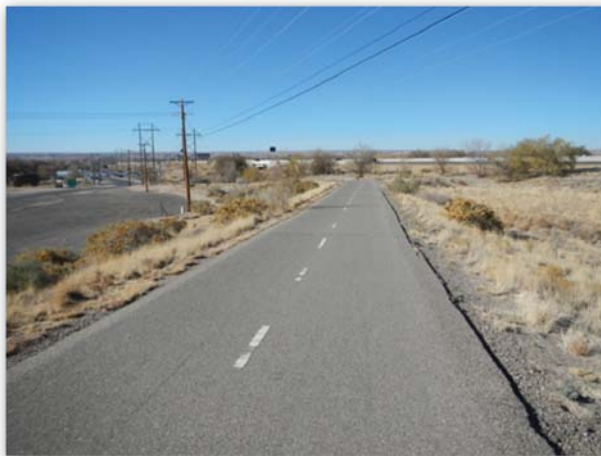
Figure 76. Segment 8, Trail edge higher than shoulder
