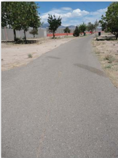
Figure 66. Segment 4, Faded centerline striping
