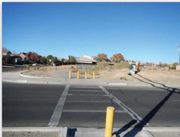
Figure 54. Segment 7, Mid-block crossing with marked crosswalk and use of bollards
