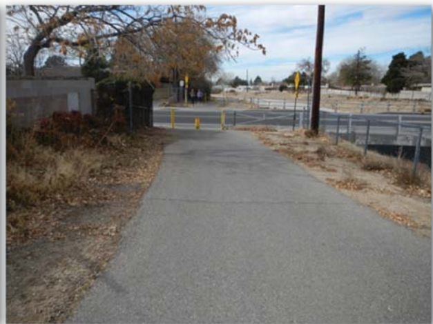
Figure 55. Segment 3, Obstructed sight distance and intersection with roadway without trail approach signing and striping
